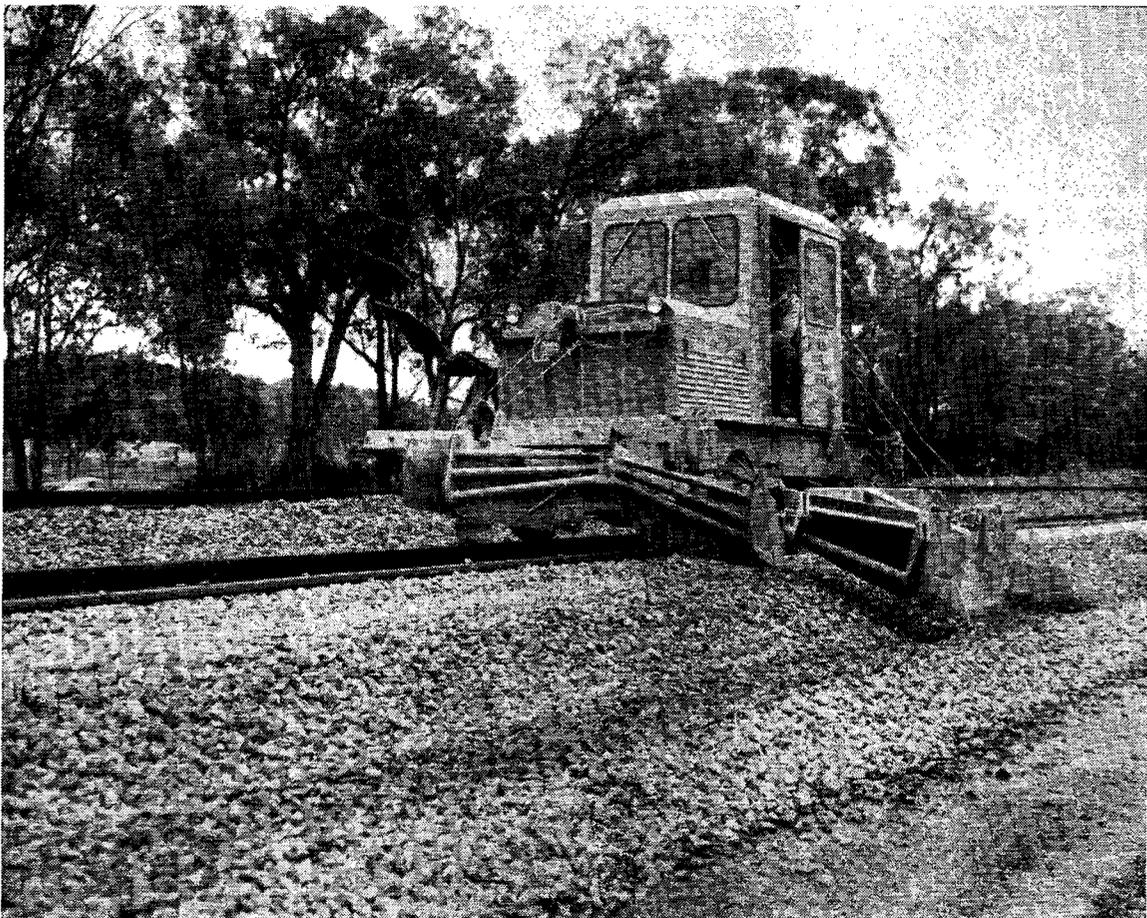
"Kershaw" Ballast Regulator operating on section of standard gauge track.
