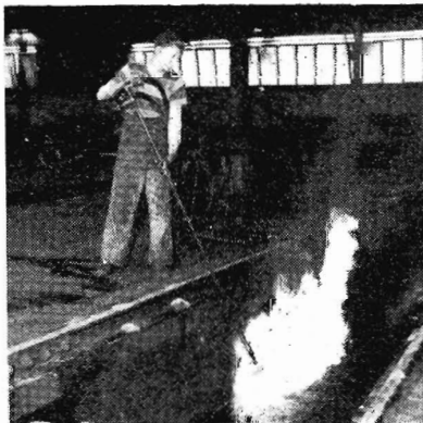
CLEANING AND FEEDING: The ash elevator (left) eliminates much of the manual work in removing ashes from the pit and loading them into trucks. The pits in the engine shed are thoroughly cleared of oil by the use of the flame-thrower, operated by Labourer W. Haberfield (centre). At right, new railwaymen B. Kirsbaums and E. Mittenbergs fill barrows from the floor of the coal stage ready to feed the locomotive tenders.
