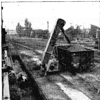
CLEANING AND FEEDING: The ash elevator (left) eliminates much of the manual work in removing ashes from the pit and loading them into trucks. The pits in the engine shed are thoroughly cleared of oil by the use of the flame-thrower, operated by Labourer W. Haberfield (centre). At right, new railwaymen B. Kirsbaums and E. Mittenbergs fill barrows from the floor of the coal stage ready to feed the locomotive tenders.
