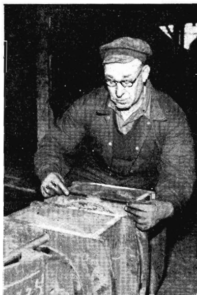
WHEELS AND AXLES: Trainee Engineman G. Schmatzko (above) cleaning tender bogies, and, below, Fitter A. Ireland marking off an axle box.
