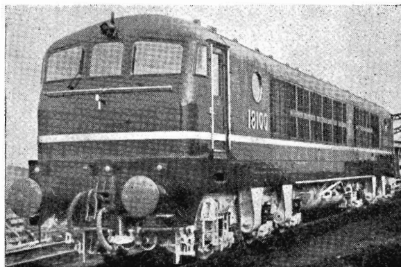
Gas-turbine locomotive, No. 18100, built by Metropolitan-Vickers Electrical Co. Ltd. for the Western Region of British Railways. It is now undergoing initial trials.
