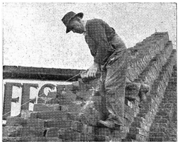
Leading-hand Bricklayer J. Prouse preparing the abutment of the Toorak-rd. bridge to take the additional structure for the double track.
