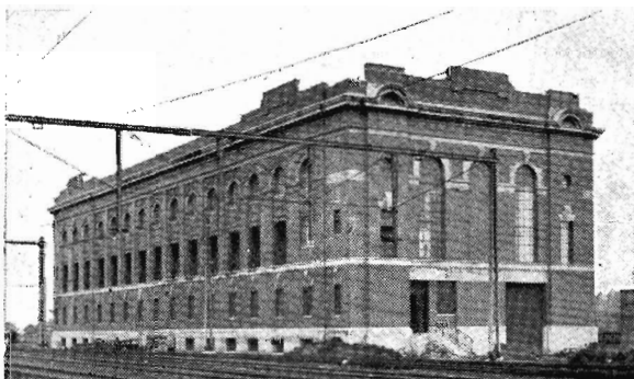
Jolimont sub-station in 1918. There are 20 other smaller sub-stations also feeding power to the suburban electric overhead wires. The sub-stations convert the 20,000 volts alternating current to 1,500 volts direct current. Four of the sub-stations have mercury arc rectifiers and the others are equipped with rotary converters.
