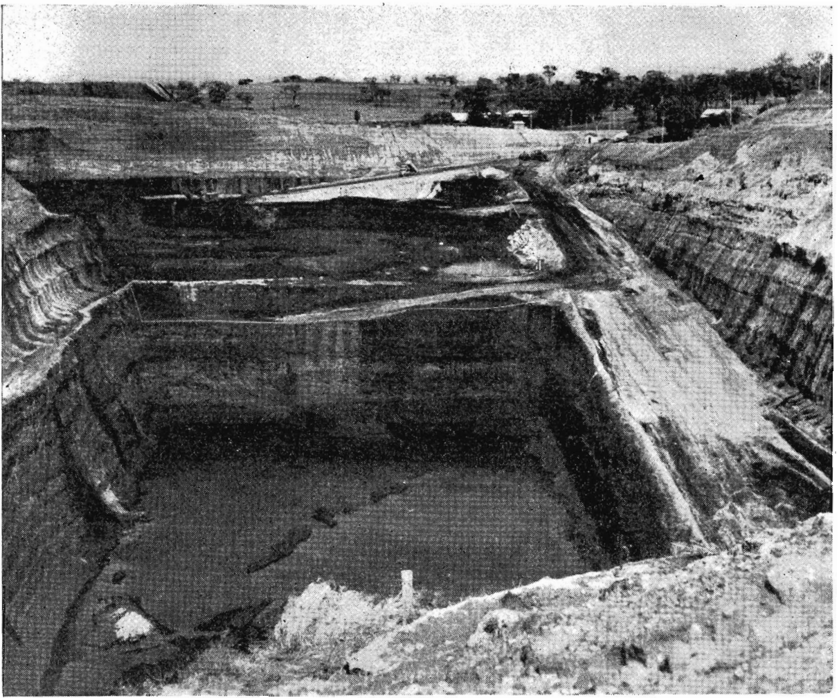
The Maddingley open cut, at Bacchus Marsh. Now in full production, it has a seam of brown coal 125 feet thick, lying under only 20 feet of overburden.
