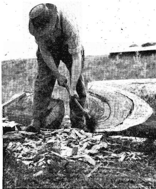
Bridge gang men are good axemen. Preparing a pile for driving.
