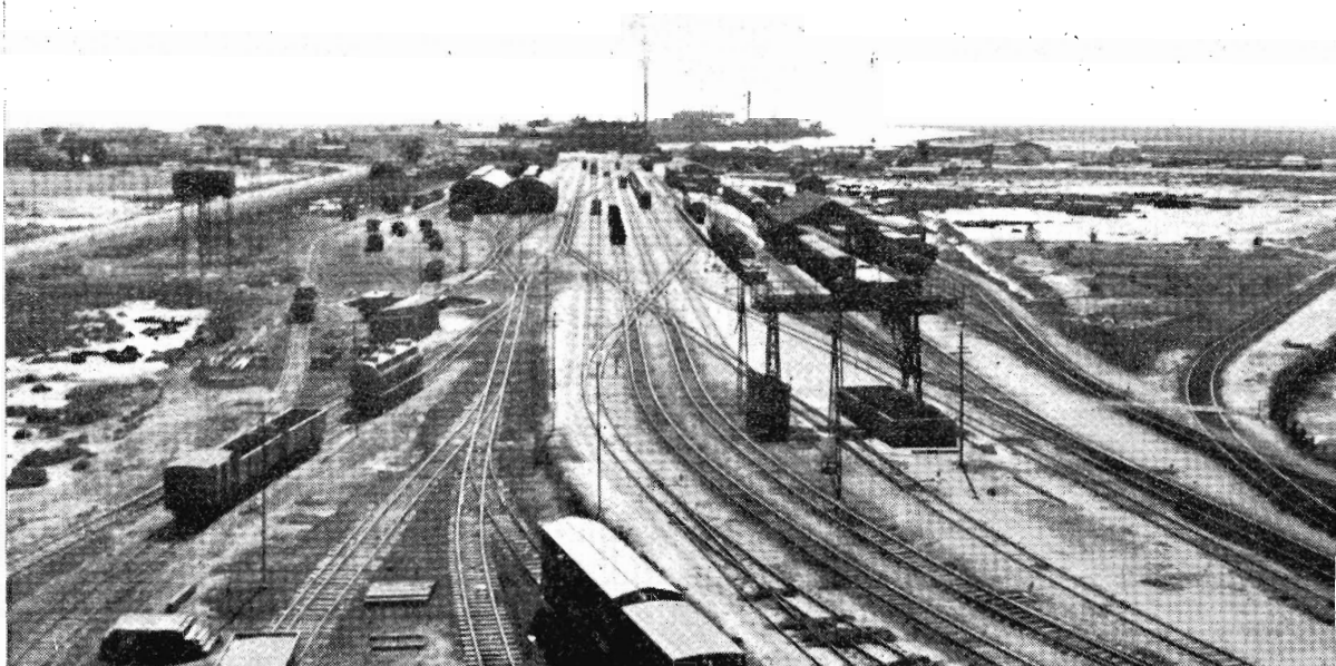
Three different rail gauges appear in this picture of Pt. Pirie, S. A. At the left and in the centre is the South Australian Railways 3 ft. 6 in. gauge, with a short section showing the third rail for 5 ft. 3 in. gauge. On the right is the Commonwealth Railways 4 ft. 8 1/2 in. gauge, crossed (at the extreme right) by the South Australian 5 ft. 3 in. track. —(Photograph: John Buckland)
