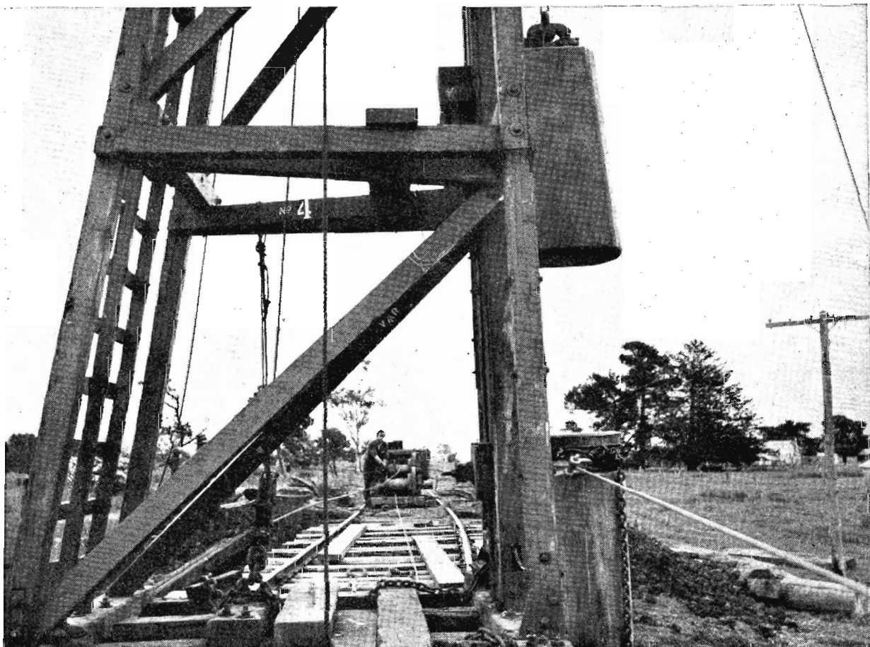
Damaged in recent floods, the timber bridge at Matthew's Creek, near Pennyroyal on the Birregurra-Forrest branch line, is being repaired. The picture shows pile driving work in progress.
