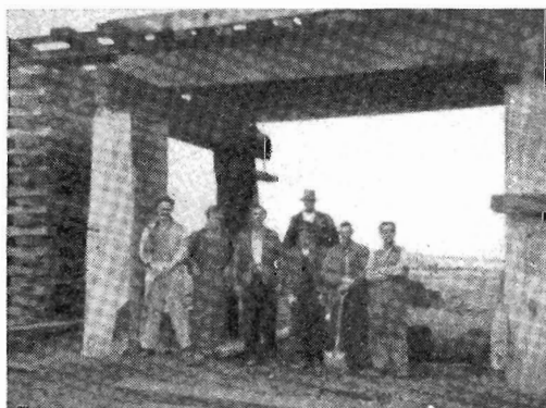
Quick restoration work followed upon the fire which destroyed 12 piles and three bays of this bridge between Gelliondale and Alberton. Forty-five feet of decking was also damaged. The fire was put out at 4.30 p.m. on Thursday, January 10. Repairs were carried out and the bridge made fit for traffic at reduced speed in time for the first train on Monday, January 14. These photographs were taken by Ganger D. Leahey, of Yarram.
