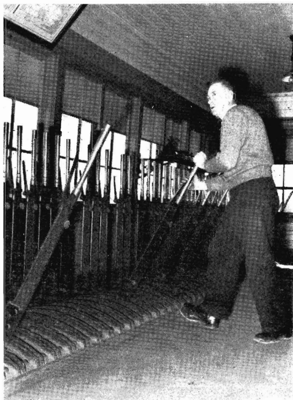
The signalman "makes a road." The levers are coloured according to their job. Black levers operate points; blue levers bring the lock bar into play, locking the points so firmly in position that a train cannot displace them; and the red levers work the signals.
