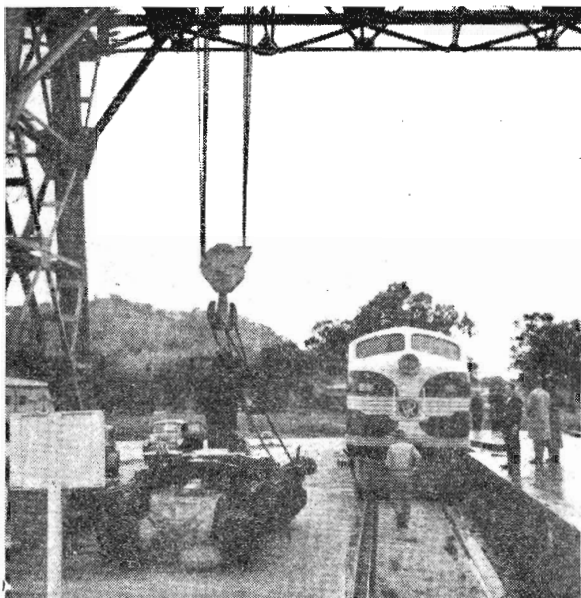
UNLOADING BOGIES : Lifting a 5' 3" bogie from N.S.W. truck prior to changing over bogies. As will be seen in the picture, three rails have been laid to enable both Victorian and N.S.W. trucks to be shunted into the platform. This facilitated the bogie changeover.
