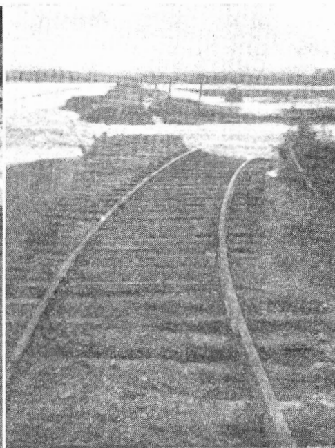
COWWARR BRIDGE REBUILT: A feature of the recent State-wide floods from the railway point of view was the excellent work done by a Way and Works gang from Sale in tackling extensive damage at Rosedale and particularly at Cowwarr where a torrent of water swept down from the Walhalla Hills, forming a new river and altering the whole appearance of the countryside. A large section of the Cowwarr bridge was swept down stream: but it was rebuilt and was fit for traffic, at reduced speeds, a little more than a month later. Above: the flood damaged bridge. Below: Traralgon-Maffra rail-car passing over rebuilt bridge.
