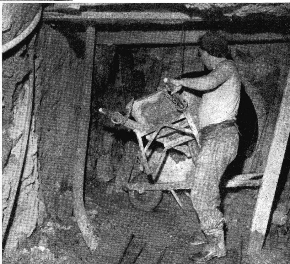
SUBWAY PROGRESS: Excavated earth being removed from the tunnel under Flinders-st. station in which pipes have been laid to carry drainage into the river. The way is now clear for the construction of the subway.
