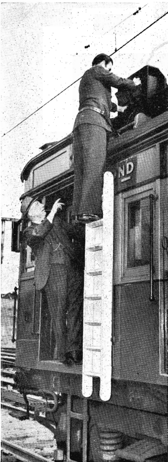
This trainee is being shown the right way to renew a main fuse on the 1,500 volt circuit and to observe safety precautions. He is equipped with a safety belt, which hooks on to the top of the car and allows him free use of both hands.
