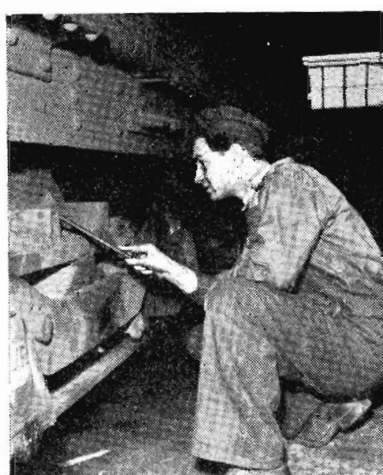
WHEELS AND AXLES: Trainee Engineman G. Schmatzko (above) cleaning tender bogies, and, below, Fitter A. Ireland marking off an axle box.
