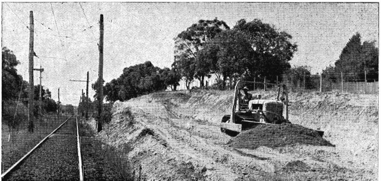
A bull-dozer scoops up the earth ready for the carry-all. Hartwell station can be seen in the background.
