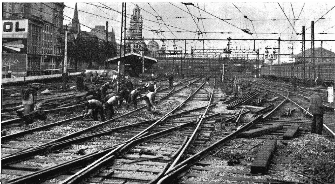
RENEWAL: Points and crossings on the busy section west of Flinders-st. station were completely renewed recently.
