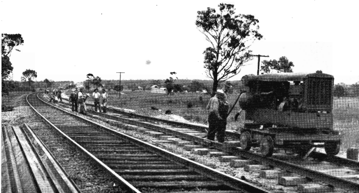
BALLASTING : Concurrently with the duplication work, the existing track is being relaid with 107 lb. rails and reconditioned with additional sleepers and ballasting. Power signalling is included in the scheme.
