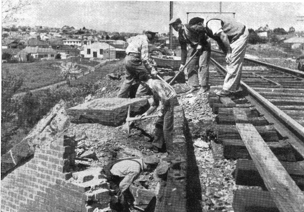
Opening up the track at Toorak-rd. bridge for alterations to the abutment.
