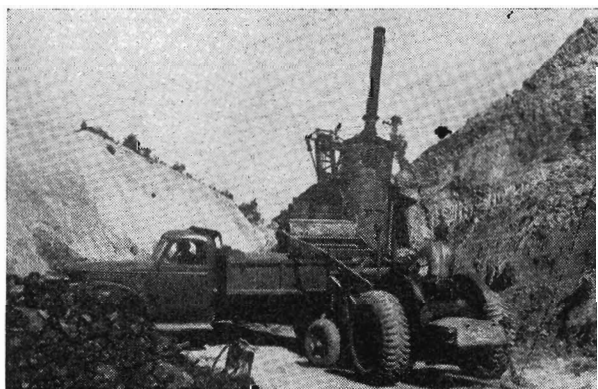
EXCAVATING A CUTTING: Steam shovel and front-end loader at work
