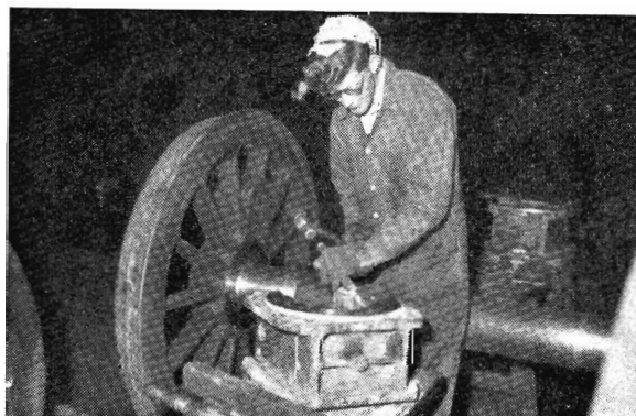
LOCO. REPAIRS: Fitting engine coupled-wheel axle box to journal.
