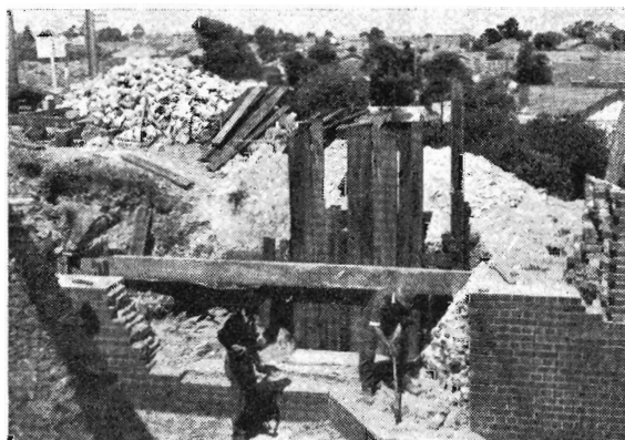
Preparing the existing abutment at Toorak-rd. bridge to take girders for the new track.
