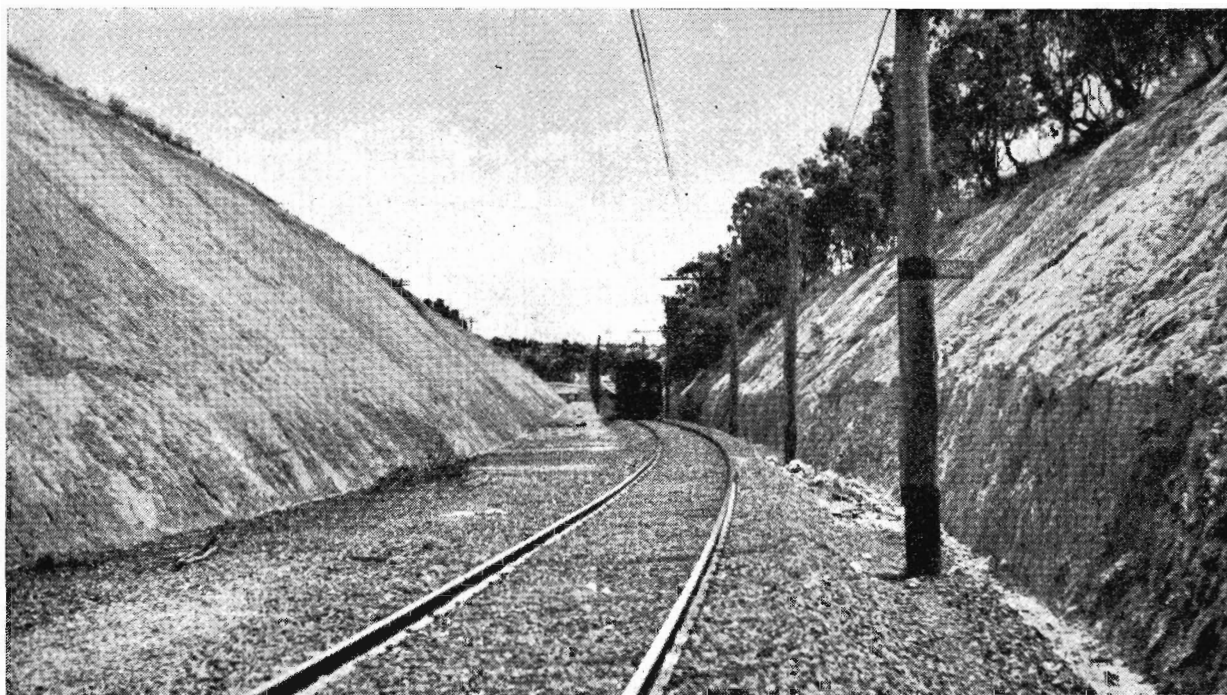
ASHBURTON LINE DUPLICATION : Earth moving equipment was used to widen the cutting for the new up track on the Ashburton line. The line of overhead masts in the distance is in the way of the alignment of the new track, and the existing wooden poles are being replaced by new steel structures. If funds are available in the next financial year, plate laying work will then begin.
