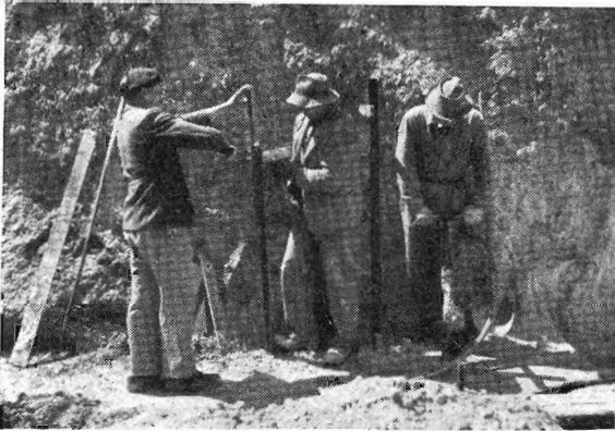
A pneumatic spade is used in excavations for the new platform at Willison station.
