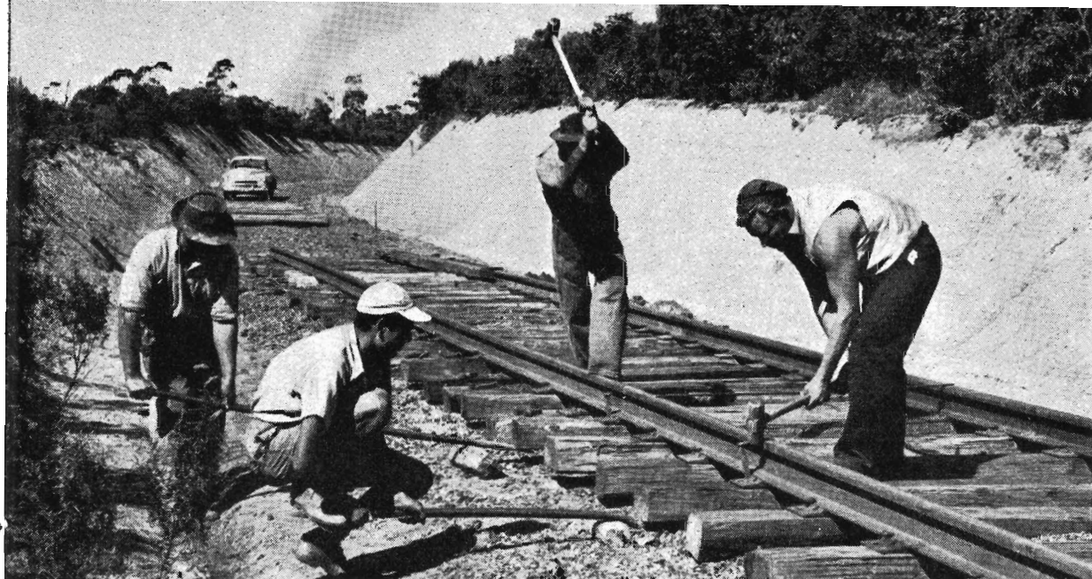
PLATELAYING: Gang gauging and spiking 94-lb. track at the head of the road, about \frac{1}{4} of a mile from Yallourn marshalling yards. Welded 135-ft. rails and sleepers are hauled by rail-tractor from depot.
