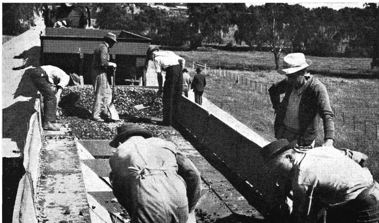
BALLAST: Discharging a QN truckload.
