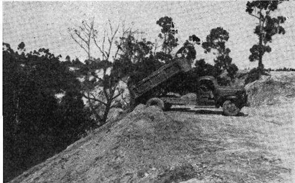
EARTHWORKS: Tipping material on bank near Latrobe River.
