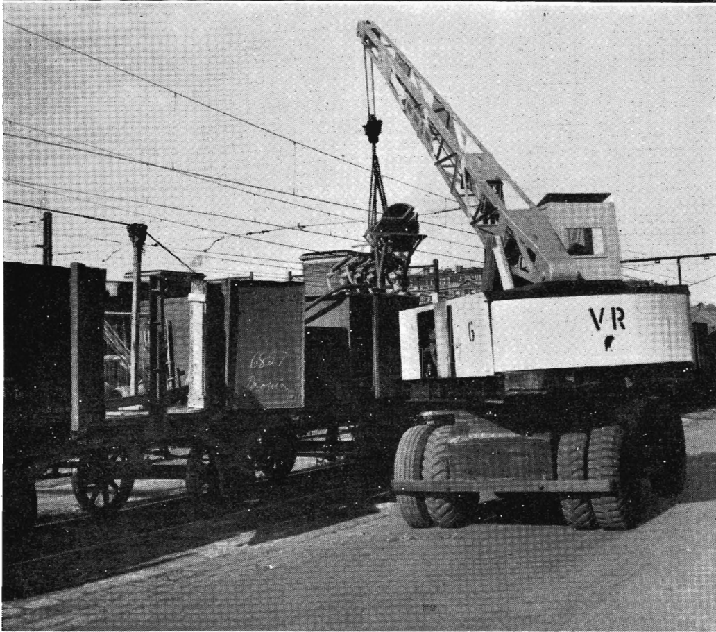
CRANE LIFT: One of the new petrol-electric cranes imported by the Department at work at Melbourne Goods. The new cranes will help to speed up goods handling.
