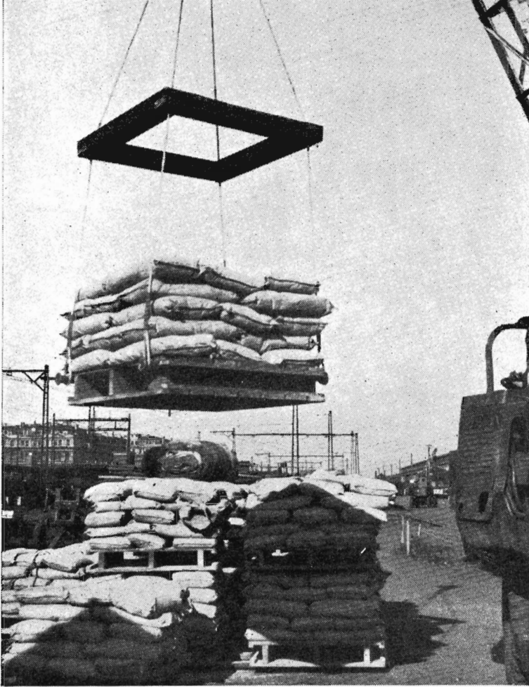
A cement handling method that was tried experimentally to make it easier and avoid damage to bags.
