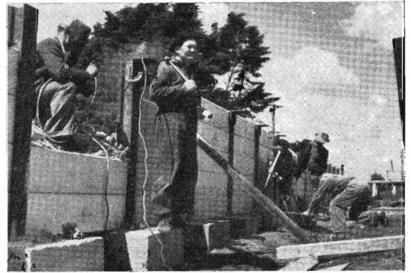
Work in progress on the new platform at Willison. Steel rails are used to support the reinforced concrete facing
