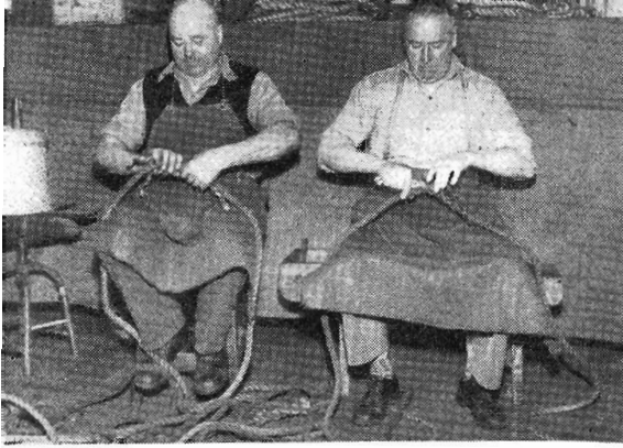
Truck lashings being repaired by Flax Splicers E. Neuman and C. Holman.
