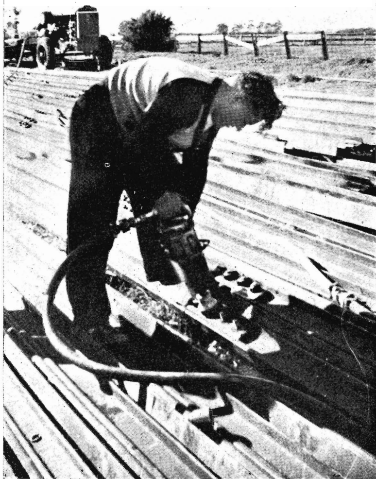
BREAKING UP : An impact spanner speeds up the job of undoing the fishbolts to separate the rail lengths. (The photographs illustrating this article were taken by Mr. F. D. Brown, Acting Special Ganger, of Korumburra.)
