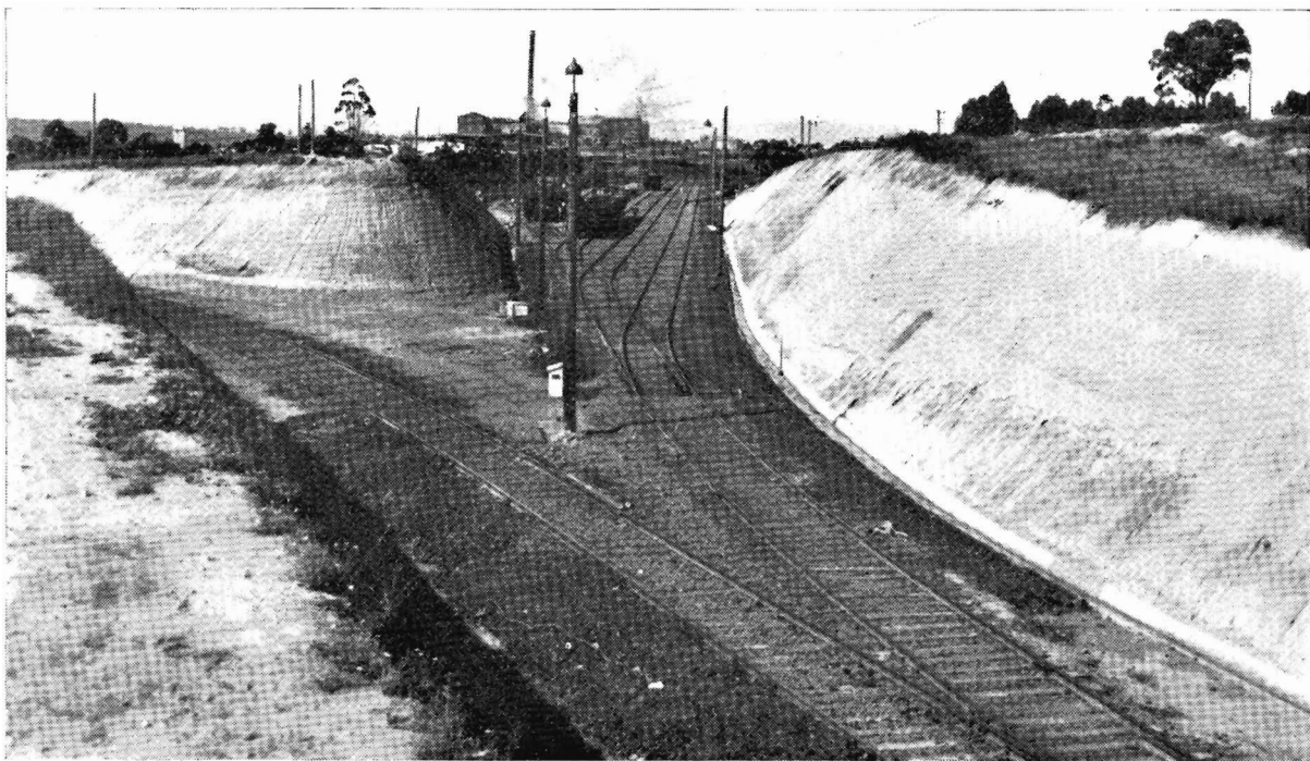
YALLOURN MARSHALLING YARD: One of the first steps taken to cope with the increased brown coal and briquette traffic was the establishment of a new gravity marshalling yard at Yallourn. A new line, a little over five miles long, with a maximum grade of one in 110, will connect Yallourn with Moe. The railways by 1959-60 may be called upon to transport a yearly output of more than three million tons of briquettes and brown coal to Melbourne. The prospective tonnage from the Morwell briquetting factories will involve an increase of seven trains daily—from 14 to 21 in each direction.
