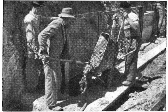
Pouring concrete for the foundations of the new platform at Willison.
