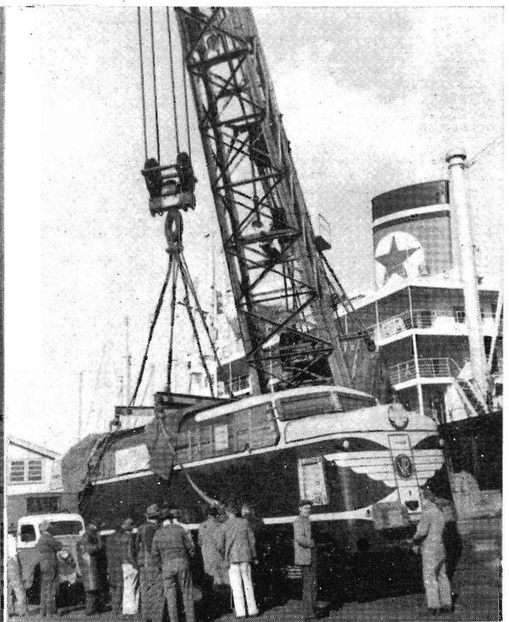
ELECTRIC LOCOMOTIVE: L1161 was lifted from the ship by a 60-ton gantry. Delivery is now at the rate of two a month.
