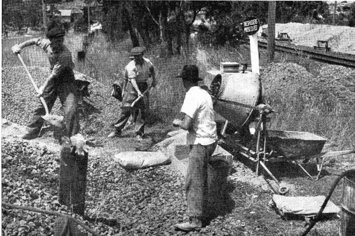
CONCRETE MIXING : A gang mixing concrete for the foundations for the new overhead masts on the Ashburton line, near Ashburton station. The concrete is poured into boxes similar to those seen in the background.
