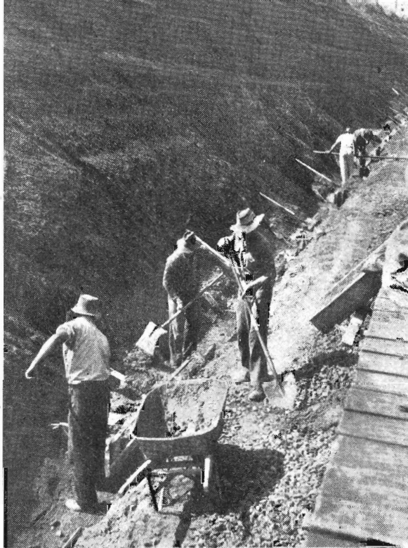
LEVELLING : The mixed concrete poured into the form work is being levelled and finished off. The plant train, on which the concrete was mixed, carried two 400 gallon tanks of water, about 300 gallons of water in drums, 100 bags of cement, and 40 and 20 yards of screenings and sand, respectively.
