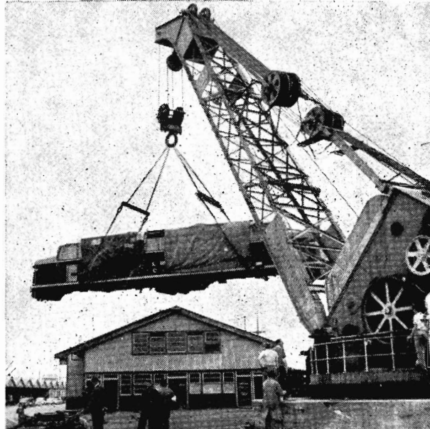
THE LIFT : After the locomotive body had been protected with tarpaulins, it was hoisted by the 60-ton crane, swung over the ship's side, and lowered to its bogies which had already been placed in position.
