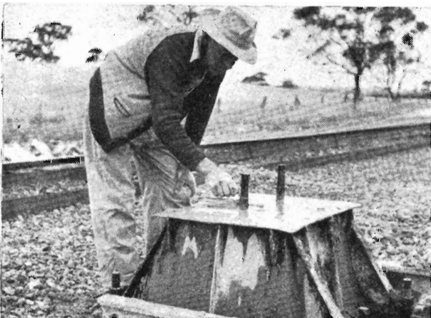
After the bolts are placed in the concrete, the finishing touches are done by hand.
