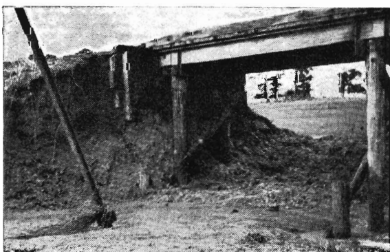
After the flood waters had subsided. Large quantities of earth were washed away from the bridge abutments during the flood.
