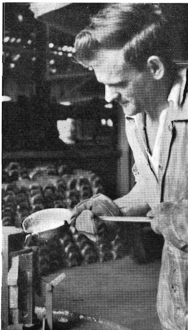
Filling the brass shell with molten metal.
