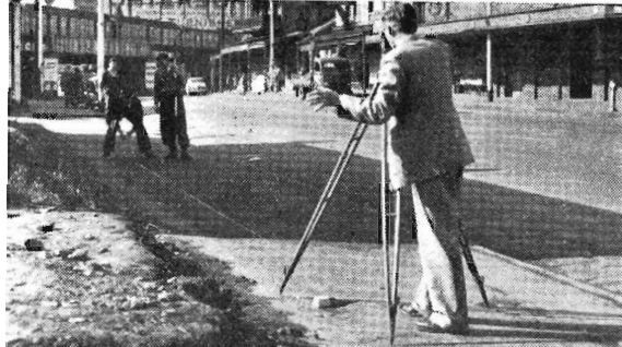
(above) Setting down base line along Swan-st., Richmond, for the rearrangement of the station.
