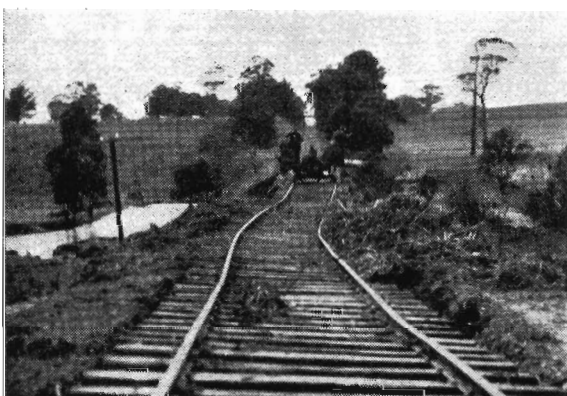
Inspecting the damaged approaches to the Barwon River bridge, where the flood waters had washed away the ballast and slewed the track out of position.
