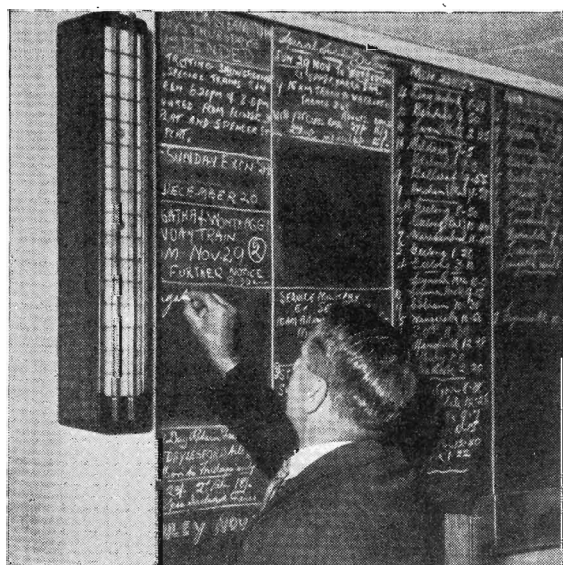
Mr. G. Cracknell enters train information on the blackboard. A direct line to Train Control enables the information to be kept up-to-the-minute. On the left is the indicator that shows waiting calls and those being answered.
