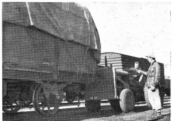
Tractors are used for shunting in goods yards.
