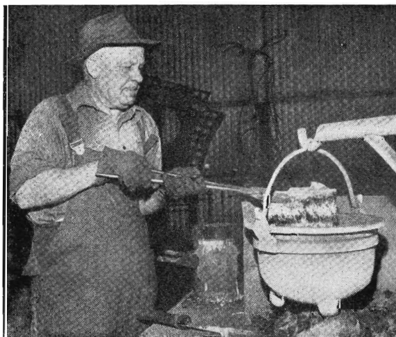
Truck axle box brasses are metallised by Metallur W. A. Beard.
