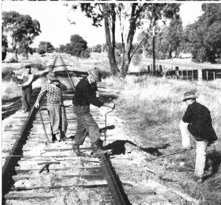
STEEL SLEEPERS : Some of the 200,000, imported from France, are being laid at Tallygaroopna.
