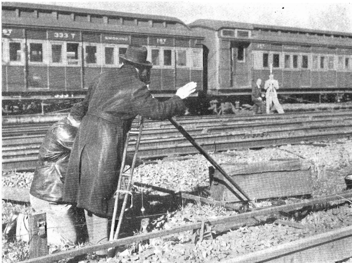
Setting line and distance to reference peg.
