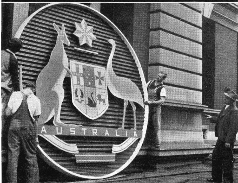
ROYAL TOUR DECORATIONS: Erecting one of the four 11-foot diameter medallions that form part of the Flinders-st. station decorations. To affix the medallions a recently developed gun was used that fires a specially shaped nail through the wooden batten into the masonry.
