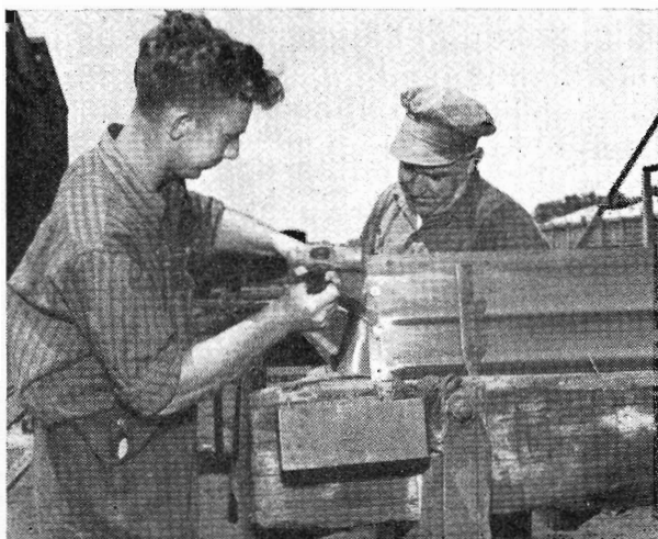
Apprentice Boilermaker R. P. Rasmussen and Boilermaker's Help L. Mahony assemble louvres prior to refitting to frame of louvre truck. At right, Stoker A. J. Purden stokes the stationary boiler which supplies steam to the workshops.
