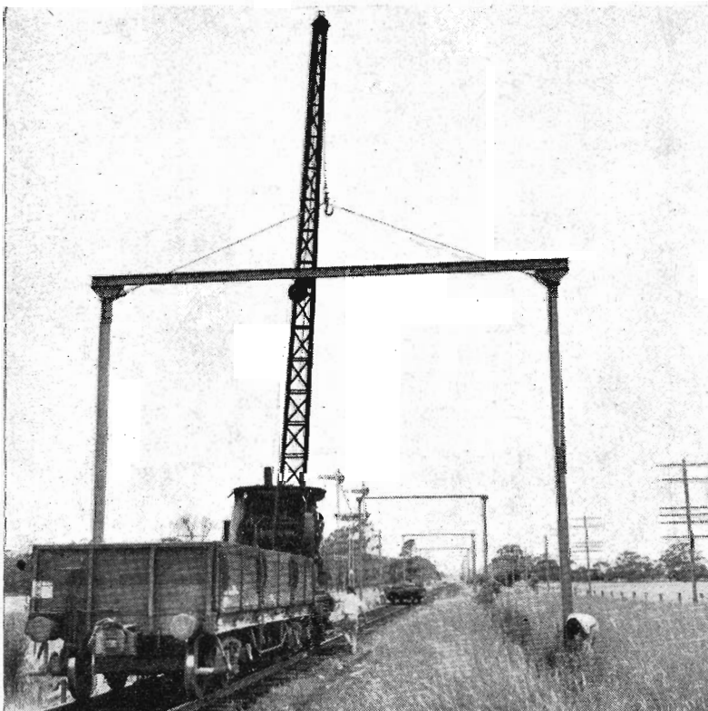
Hoisting the overhead structure to its foundations. A line of completed structures can be seen in the background. This particular section of track has not yet been duplicated.
