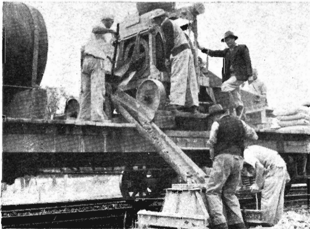
When the foundations are close to the track, the concrete is poured direct from the mixer through a metal chute.
