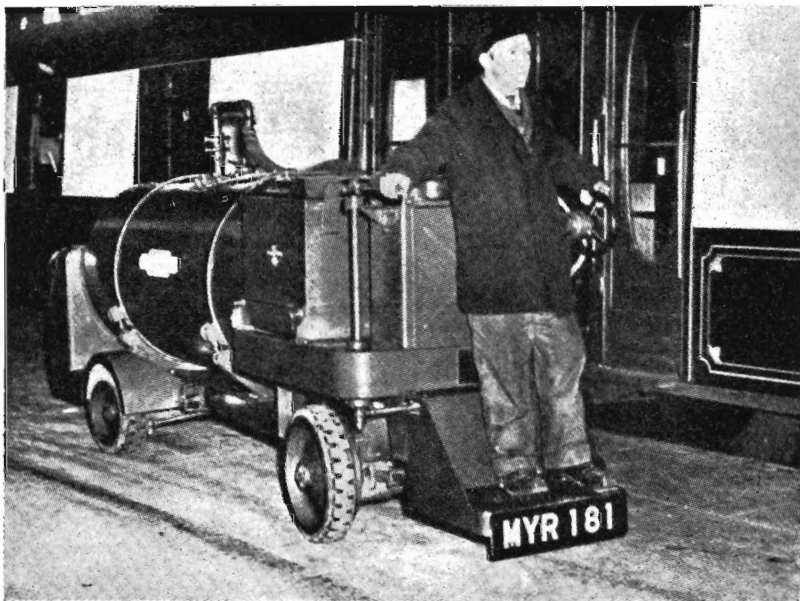
Battery operated water tank of 275 gallons capacity, used by British Railways to replenish the water tanks of long-distance passenger rolling stock.
