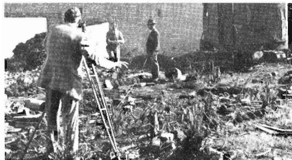
(below) Setting out alignment of new tracks at the rear of Richmond station.
