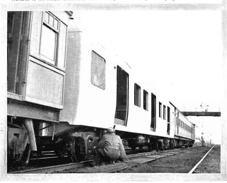
TEST RUN: One of the new suburban cars was recently tested on a run between Melbourne and Werribee. The Acting Chief Mechanical Engineer (Mr. G. F. Brown) is here seen making a bogic inspection at Werribee.
