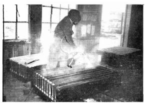
Spraying moulds with oil.
