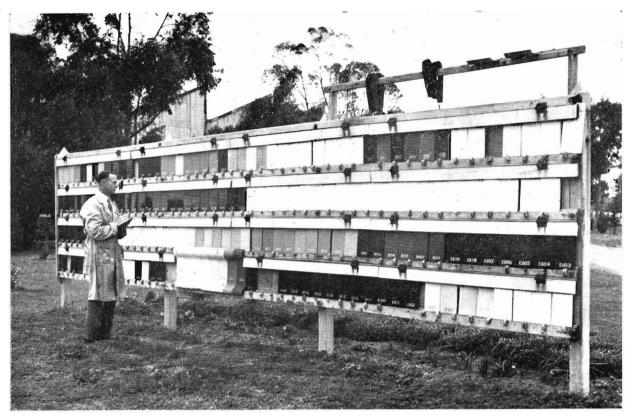
Exposure board for testing paints in outside weather conditions.
