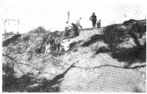
The timber bridge at this spot on the Glen Waverley line has been replaced by a large concrete pipe for drainage.
