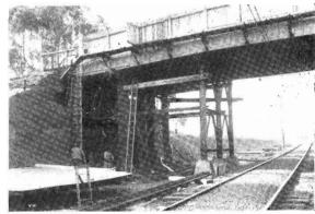
The new down track at Mt. Waverley, on the Glen Waverley line, will pass through the widened opening of this bridge.
