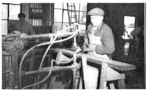
Welding reinforcing wire into shape.
