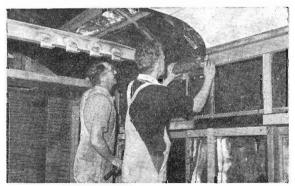
Installing body packings.
