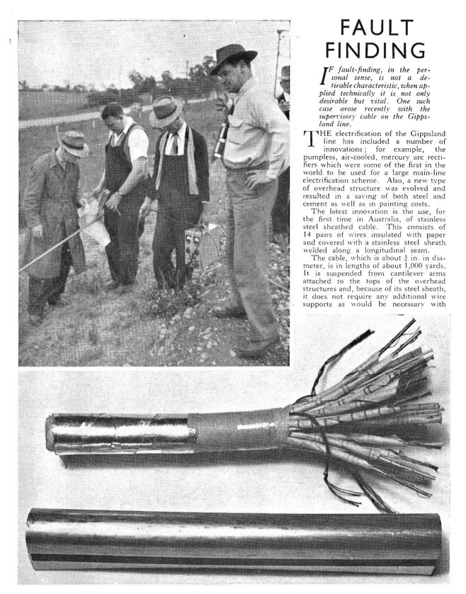
Looking for the fault (top). A piece of rag is used to shield the probe of the detector unit from the wind. Below is the core of the cable (with some of the insulation removed to show the actual conductors and the method of insulation) and the stainless steel sheath.
