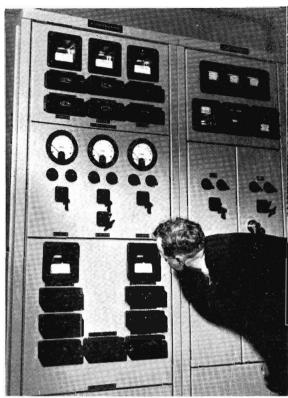
Assistant sub-station electrician M. Gorson inspects a "Translay" relay on the feeder control panel.
