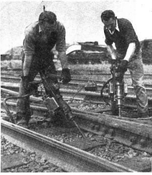
(Left) Gang re-gauging crossing work. (Right) In the confined spaces at crossings, mechanical tie tampers are particularly useful for sound packing of timbers.
