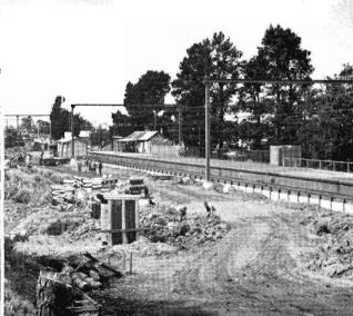
GIPPSLAND LINE: New station yards and a platform for a second track are being built at Garfield.
