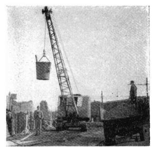
A dragline excavator being used as a crane to remove earth for the foundations of the retaining wall.
