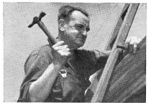
A Works Foreman's plumber repairing spouting at a suburban station. The plumbers are given a district in which to work. Their routine jobs include repairs to roofs and spouting of station and workshop buildings.
