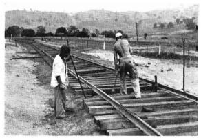
Platelaying near the start of the second deviation.
