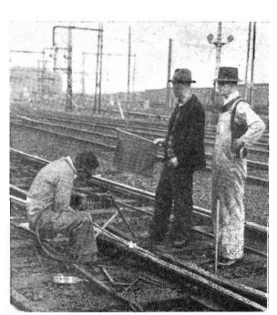
Welder surfacing a worn crossing near Spencer-st. Repairs to the average worn crossing might require from 200 to 300 cubic feet each of oxygen and acetylene, and about 4 lb. of alloy steel.
