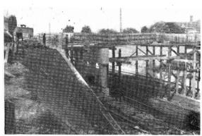
The track leading to the flyover will pass under the reconstructed Stanhope-gve. bridge, Camberwell, between the pier and abutment (left).
