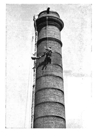
Steeplejacks repainting the steel bands around the chimney stack at Bendigo North Workshops.
