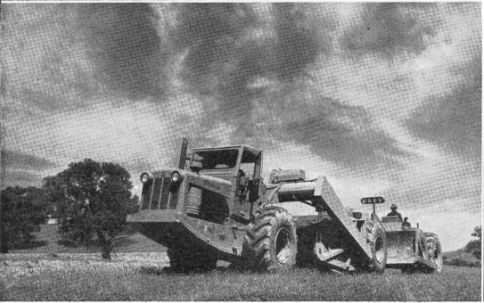
RESERVOIR ENLARGEMENT: A 15 cubic yard tractor-scraper beginning the earth works for the new Bonnie Doon station. The line is being deviated for a bigger Eildon reservoir.
