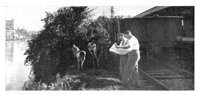
The first practical step was to raise the 20,000 volt cables on the river bank, opposite the St. Kilda platform, to make room for a barrel drain to run from Flinders-st. under the station building and empty into the river. It replaced the main drain through the area now occupied by the subway.
