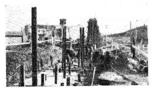
With the foundations completed, the next stage of construction is the erection of the framework for the retaining wall.
