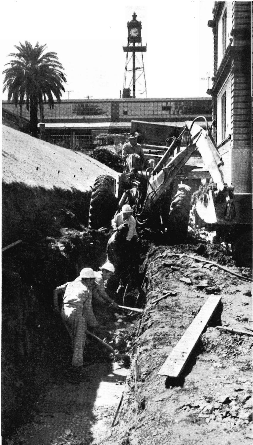
Blasting shattered the peace of the pigeons that live at the rear of Head Office as the channel and tunnel for this drain were cut. The drain, 1,516 ft. long and up to 20 ft. deep in parts will provide drainage for the new Spencer Street station and subway. It was necessary to cut 200 ft. of tunnelling, part of it through the embankment at the rear of the offices.
