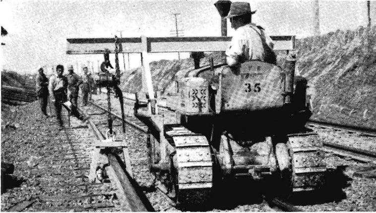
Crawler tractor, with rail threader suspended from beam, lifts rail to centre of track.
