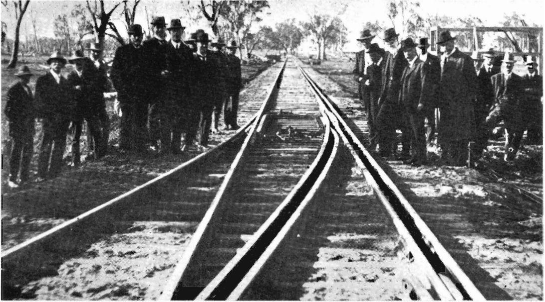
**Test at Tocumwal :** To overcome the break of gauge various inventions and expedients have been tested, but found to be impracticable. Shown above is a test of the third rail system at Tocumwal on November 12, 1915. (Photograph was sent to *News Letter* by Mr. J. M. Eaton, formerly Yard Foreman at Seymour, now retired.)
