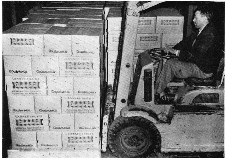
**THEY'RE STUCK!** Foods in cartons—such as tinned fruit and condensed milk—are now being carried in pallet size loads, as shown above. The cartons are held together by a special adhesive, in such a way that they are resistant to train movements but can easily be separated on arrival at destination. Each pallet load of tinned fruit weighs just over 1½ tons. This method eliminates the steel strapping of cartons at factory and also facilitates handling of goods in transit.
