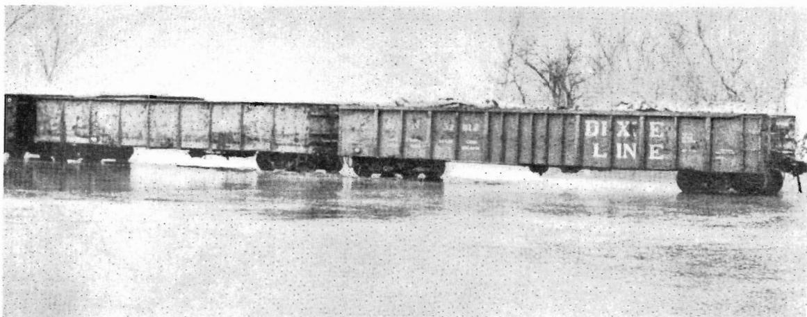
**SAVING BRIDGE:** When the Louisville and Nashville Railroad's bridge over Beargrass Creek (U.S.A.) was almost entirely submerged by flood waters, these wagons loaded with scrap iron were placed on the bridge to anchor it in position until the water had subsided. (*L & N Magazine*.)
