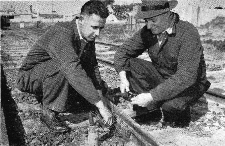
**TESTING :** Electrical Fitter-in-Charge J. D. Morelli (left) and assistant R. McLure, of Traralgon, check the insulating block joint between adjoining track circuits. This is done by connecting rail joints in a circuit with dry cell ; any leakage is revealed by deflection of a voltmeter needle.
