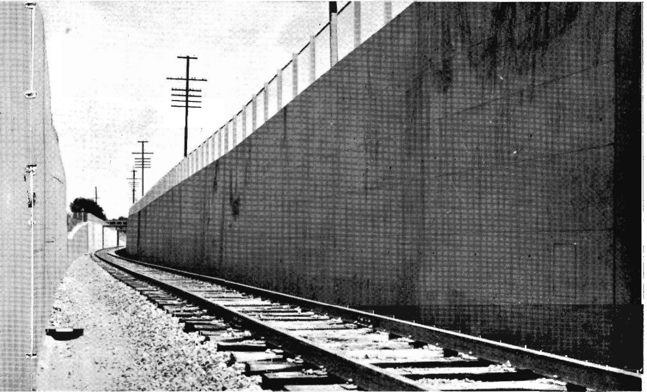
(Above) Due to the confined conditions, this 18-ft. deep cutting was necessary at Wangaratta to get the standard gauge track through the station. The cutting is 2,800 ft. long, required 55,000 cubic yards of excavation and 6,500 cubic yards of concrete for lining the walls.
