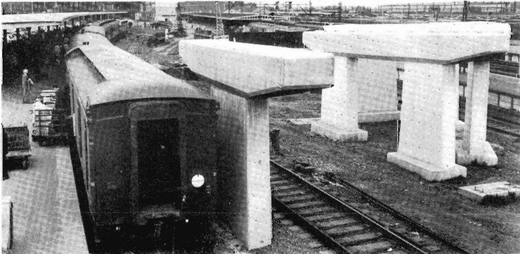
Concrete piers and cross-heads for the vehicular overpass leading from the inner car park to Spencer St.
