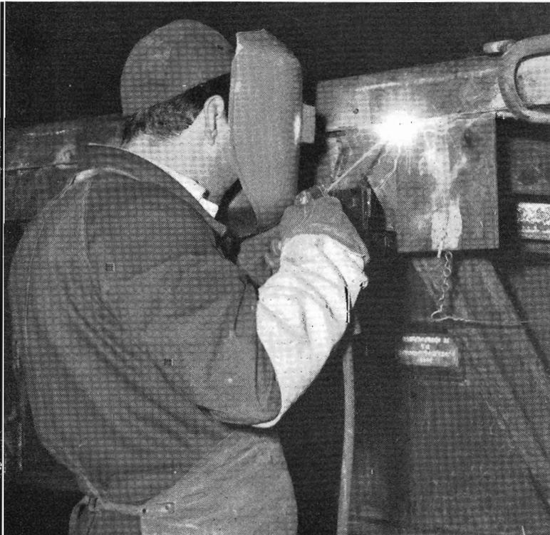
Arc welding bracket to underframe of Flexi-Van wagon.
