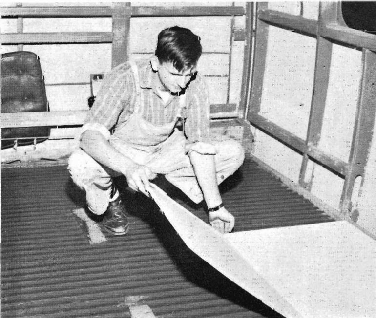
Rigid urethane foam is now being used instead of corkboard for the underfloors of *Harris Trains*.
