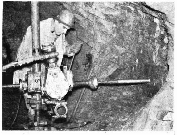
*Flat Jack Test 1* ; Operator prepares to cut slots in rock by boring a series of holes.
