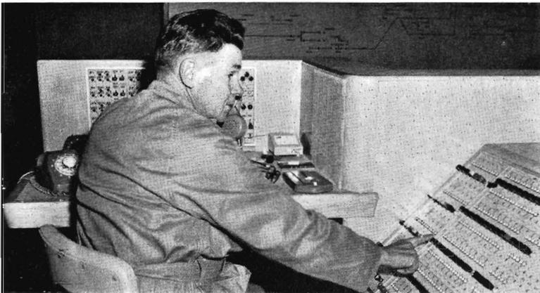
Electrical Operator W. McNamara using one of the direct lines to sub-stations and tie stations.
