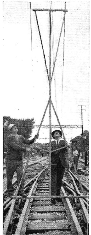
At Hawthorn, overhead staff check the stagger of the contact wire. The staggering prevents uneven wear of the contact strip on the pantograph.
