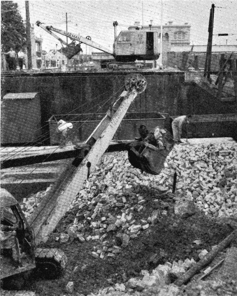
Removing debris from the dismantled bridge at Coppin Street. The street has been closed to road traffic while the new bridge is being built.
