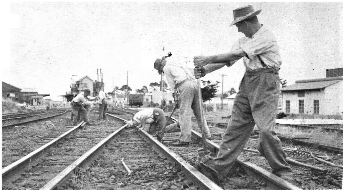
At up end of station, No. 9 gang (Ganger C. A. Vallence) lift crossing for replacing timber.
