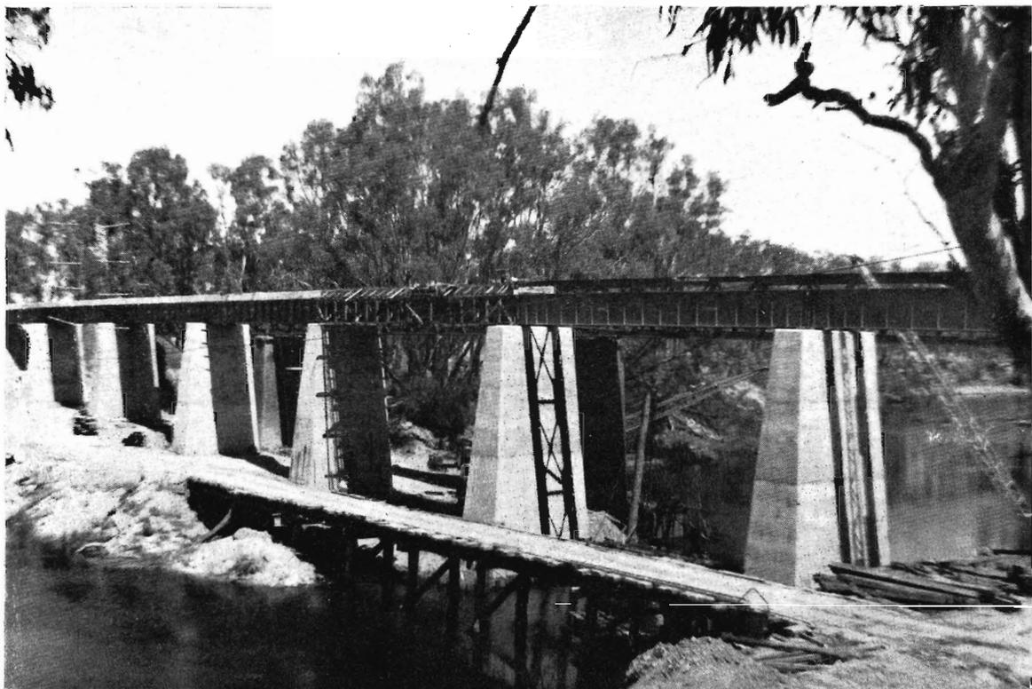
New Toolamba bridge near completion. In foreground is the temporary timber bridge that allowed plant to be quickly moved to either side of the river as required.
