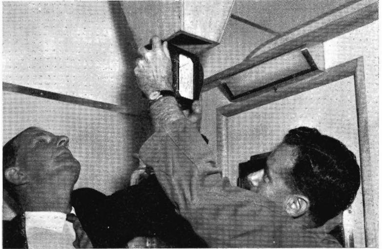
Using a velometer, Engineer H. Robinson (*left*) and Assistant Engineer W. Hoole check air flow. The pyramid shaped box is placed over the ceiling panel to measure the amount of air coming into the compartment from the air-conditioning unit. The velometer measures the velocity of the air.
