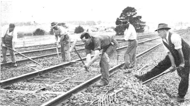
No. 10 gang (Ganger F. Law) are replacing a sleeper on down side of station.
