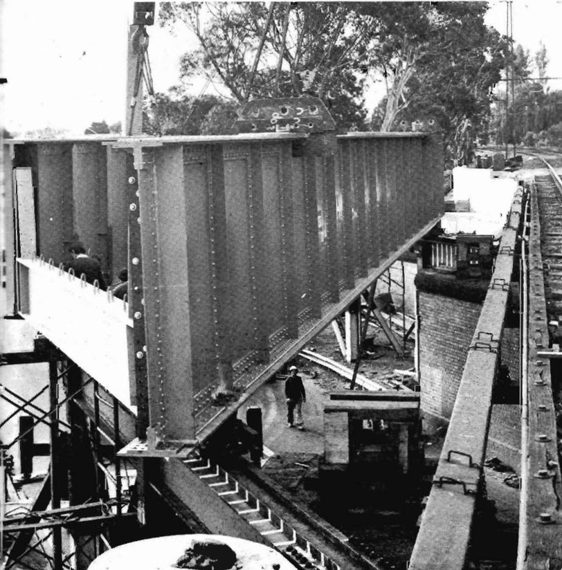
ROLL - IN BRIDGE. Nepean Highway widening works at Gardenvale entailed completely new steel work for the rail bridge. The new bridge was assembled alongside the old one, to be then rolled in to position.
