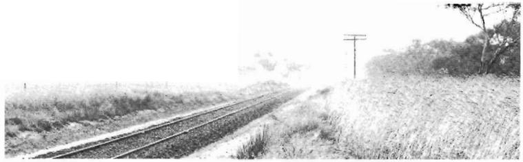
One of the pilot stabilisation plots showing how the crops are planted right to the edge of the formation.
