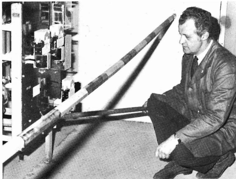
Evan Beach points to the modified control panels. Blank area shows where contractors have been replaced by diodes (visible at back of panel, tap shaped).
