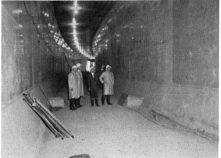
In a few years, trains will run through this area. A party from the concrete industry inspect progress on the project; the reinforced concrete walls are two feet thick on sides and top, and three feet thick at the base. Top to floor is 19 ft. and floor level at this point is 20 ft. below sea level.
