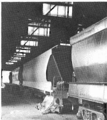
In the paint shop, wagons go through the following stages over the three days (from right): de-oxidize, primer, undercoat, finishing coat.
