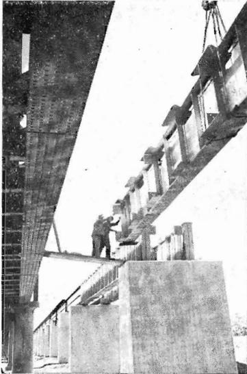
New bridges were built for the standard gauge line Wodonga and Broadmeadows. Clearly showing the changes in designs from the 1873-built broad gauge (left), is the new bridge for the 4 ft. 8½ in.
