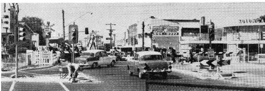
**NEW STYLE BOOMS.** The recently installed boom barriers at Clayton Road, Clayton, are the first in Victoria to have normal traffic light signals instead of large flashing red lights. The traffic lights normally control traffic at the intersection at the crossing, but when a train approaches, go to red for traffic crossing the lines, and the booms lower. Turning traffic then has the green light.
