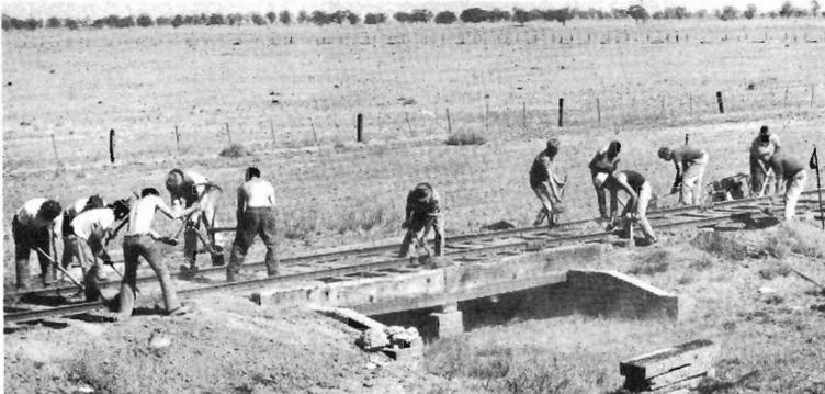
It's dry and dusty in the drought affected areas, and relaying a railway is heavy work. Presently, the 44 miles between Echuca and Denilquin is being resleepered and sledged in preparation for the relaying gangs. The Echuca Points and Crossing Gang plus the Utility Gang, and swelled by workers on drought relief, are seen here preparing the track for sledding just south of Moira station. The effect of the drought is obvious—this photo was taken at the end of October.
