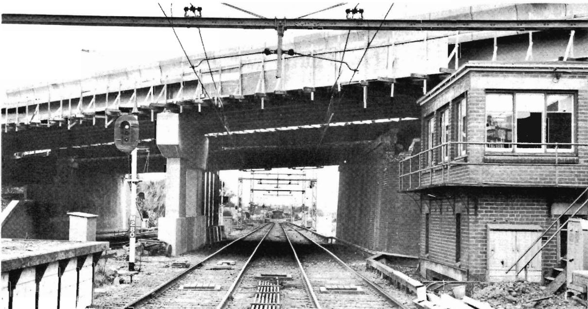
**ROOF ROAD.** Road widening works at the West Footscray overpass of Geelong Road, (known to locals as Mount Mistake) encroached on the railway signal box area. Rather than move the box, the tiled, gable roof was whipped off, and a flat roof provided.
