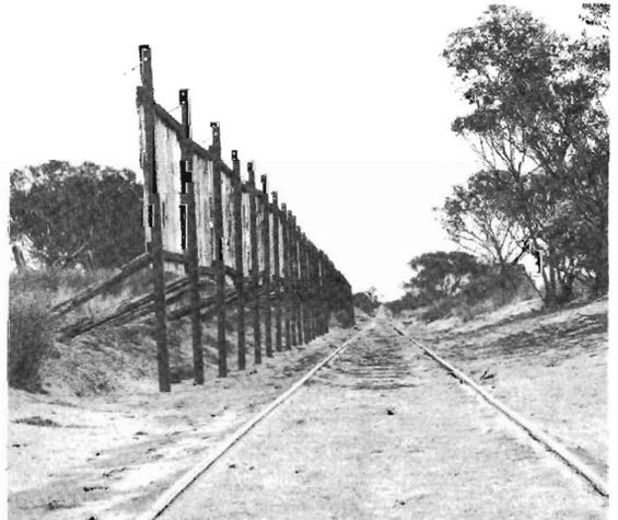
The effectiveness of wind chutes in limiting the drift accumulation on the rails is demonstrated near Pier Millan.
