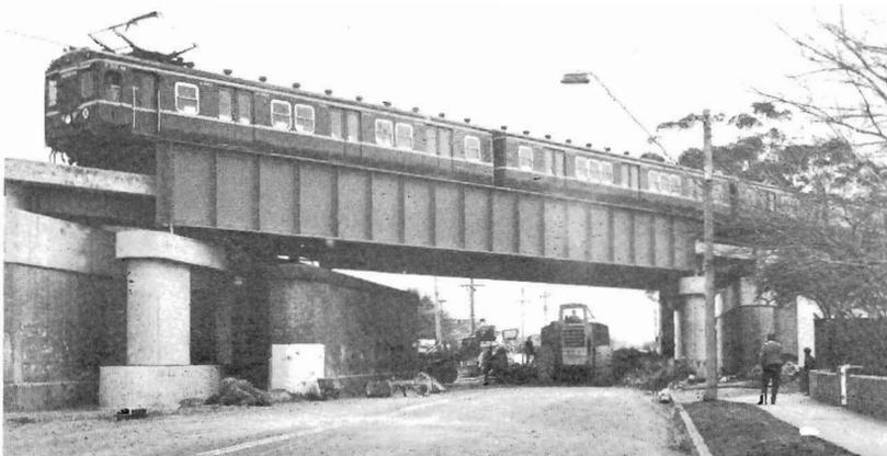
Bridge clearance has been raised, and with the other pier removed, road width will have been increased, too.
