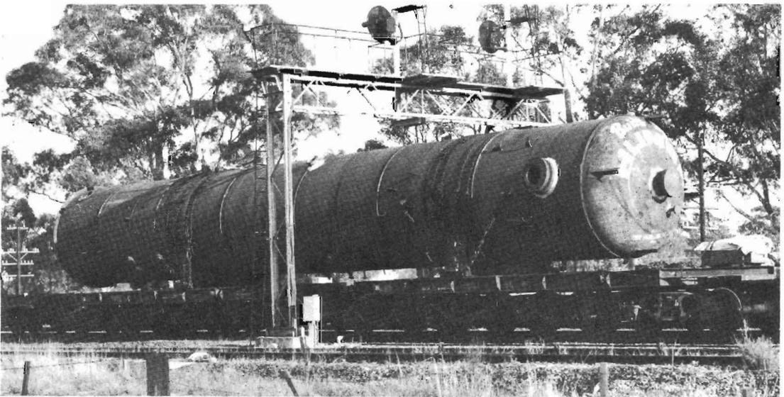
**BIG HAUL FOR BIG LOAD.** More than 1,300 miles of rail travel was in store for this huge absorber vessel bound for the Gidgealpa oil and gas field in outback South Australia. The 140-ton vessel was travelling from Melbourne to Telford, S.A., via Albury, Parkes, Broken Hill, Peterborough and Port Augusta to avoid transfers - this route is standard gauge all the way. The vessel was photographed at Violet Town on September 4.
