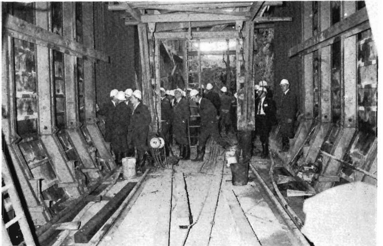
Railwaymen and other members of the Industrial Mobilization Course inspect formwork for the concrete in one of the tunnels.
