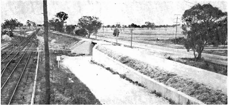
Whenever possible, and appropriate, the new standard gauge line was grade-separated. At Springhurst a flyover takes the line over the station access road.
