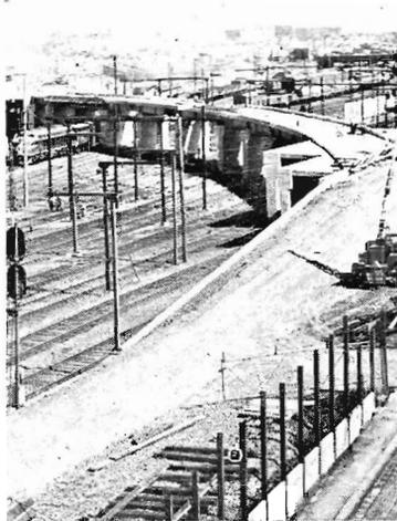
Because the standard gauge line uses the former metropolitan goods lines into Dynon for its approach to Melbourne, a new route into the city terminal, crossing the entire Melbourne Yard arrival area and western suburban lines, had to be found. A 13-pier curving concrete flyover brings the line into correct position for the run into Nos. 1 and 2 Platforms at Spencer Street.
