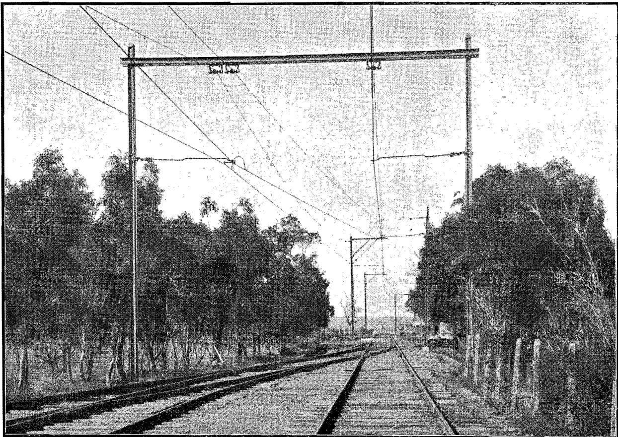
NEW TYPE OF OVERHEAD MAST STRUCTURE MANUFACTURED FROM OLD RAILWAY RAILS.
