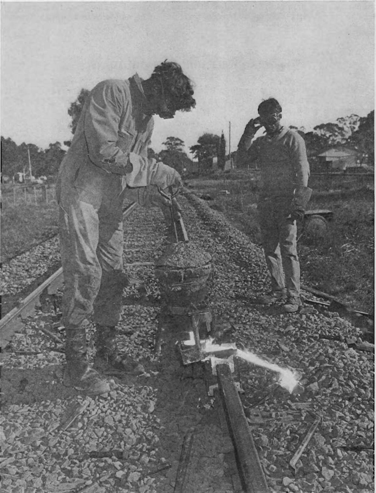
Thermit welding on the standard gauge track between Melbourne and Albury.
