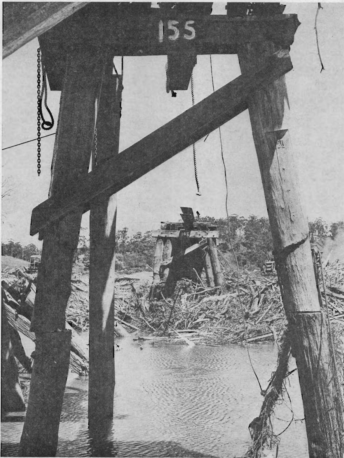
Flood damage at Orbost where six bridge piers were washed away.
