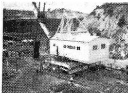
Enclosed please find snaps of a Bucyrus electric power shovel on its way to the Yallourn North Brown Coal Mine (one snap is the shovel itself). It is travelling under its own power, and you can see the high tension cable dragging behind it. The car and oil-tanker in the foreground give some idea of its size.
