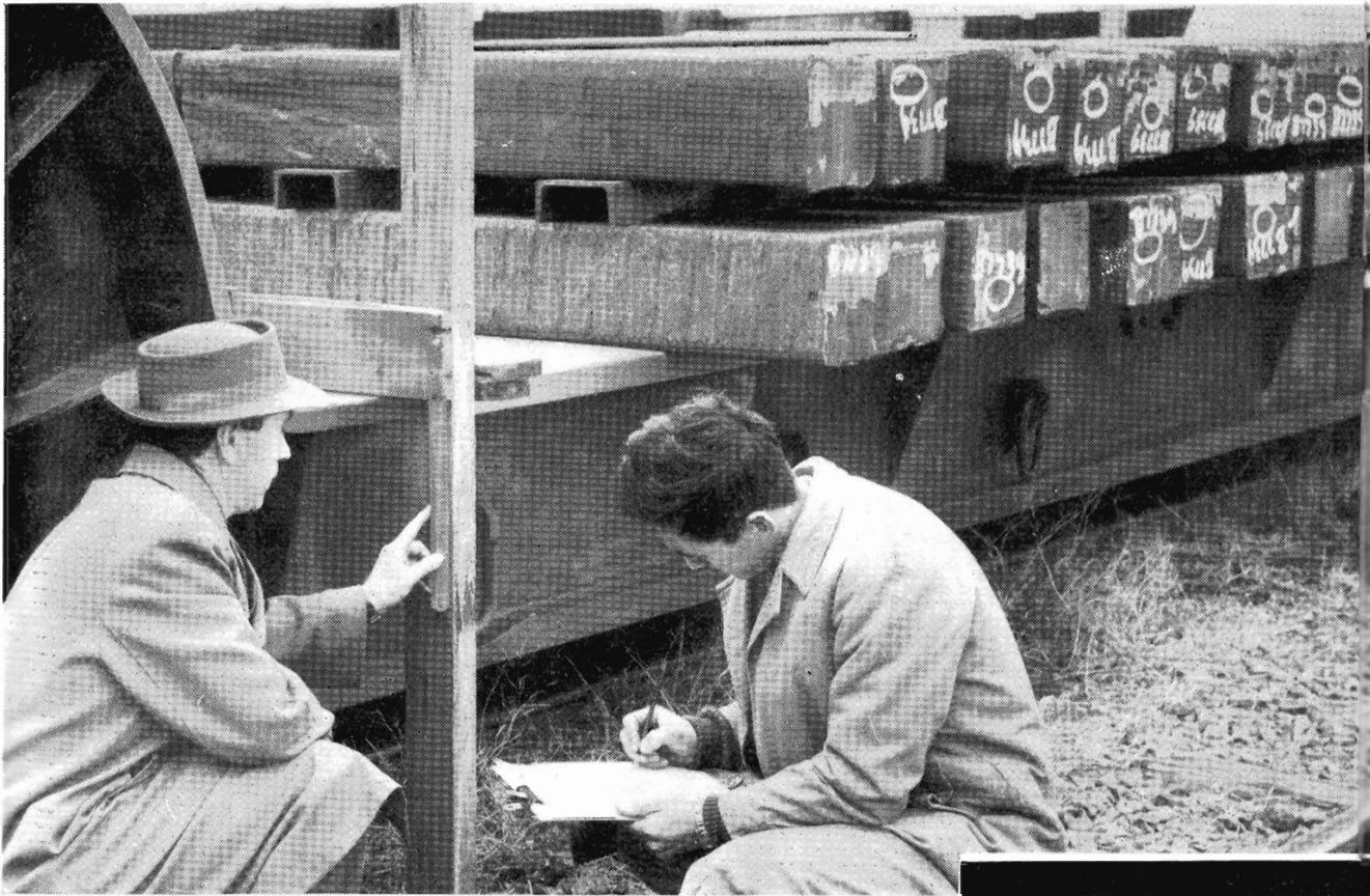
Rolling Stock Branch Engineers G. McMahon and N. Hill checking deflection, under load, of well wagon that is nearing completion at Newport Workshops. Designed to carry massive stators for the State Electricity Commission, as well as other special loads, the wagon will have a capacity of 150 tons and is the biggest of its type ever built by the Department.
