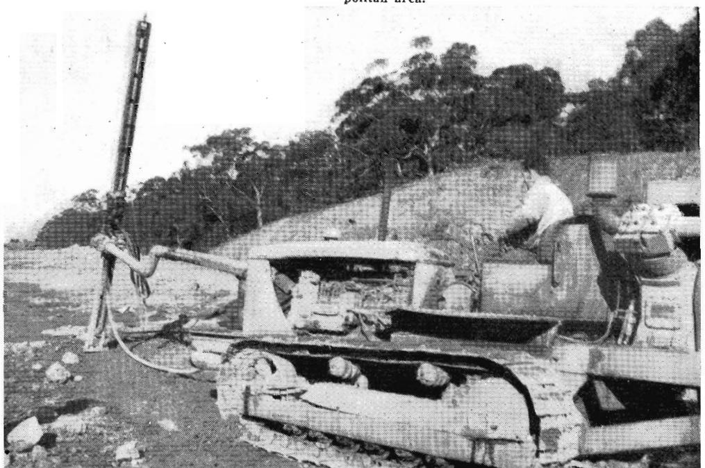
First ever used on the V.R. system, this air-driven rock drill—crawler-mounted with a forward boom for manoeuvring the drill into position—is helping between Wandong and Kilmore East to accelerate the standard gauge earthworks.
