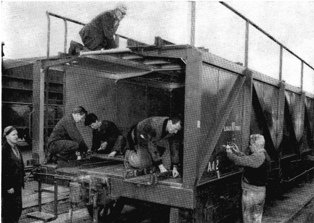
IMPROVED AA wagons for transporting motor cars have two special features: sides to obviate dust damage to cars and a roof totally enclosing the lower deck, so forming a floor for the upper deck that prevents oil dripping on to cars beneath. (Above) Fitting a wagon with motor car fastening gear. (Right) Twenty-four cars are loaded on these four AA wagons.
