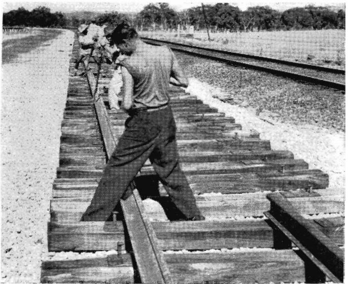
(Above) ROLLING rails into position on standard gauge track near Bowser. Scheme requires about 27,000 tons of rails, 450,000 sleepers, 600,000 cubic yards of ballast and 2,800 tons of steel for bridges.
