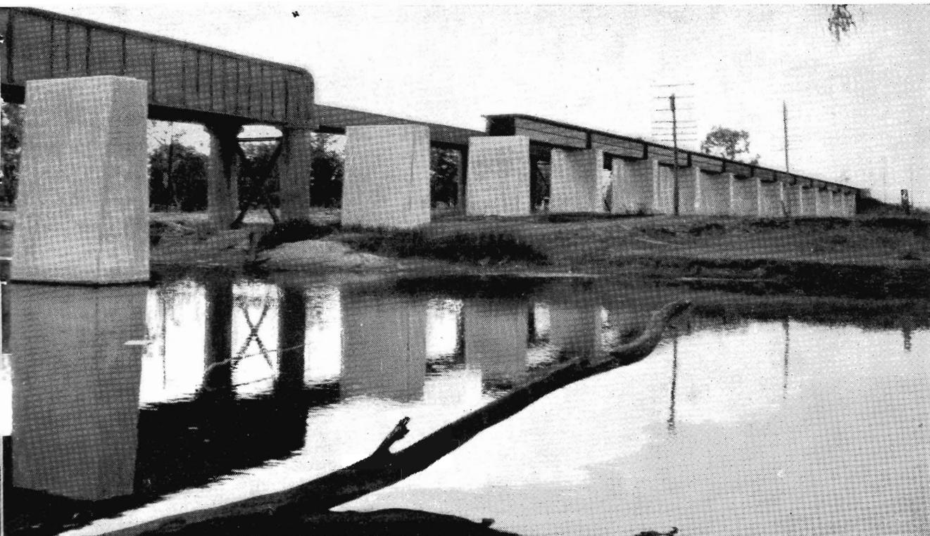
**BRIDGE** over Broken River, near Benalla. Concrete piers at the right will take standard gauge line. Steelwork on the approach spans (supplied by N.S.W. Railways) has been erected. The river spans are 63'; plate girders are now being fabricated for these.
