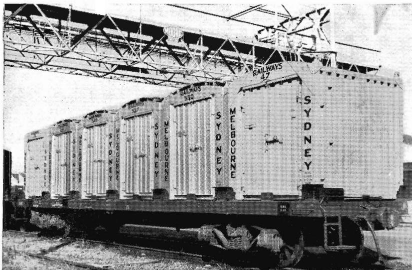
Steel containers exploit the inherent advantages of each form of transport—road for local pick-up and delivery, and rail for long-distance bulk haulage.
