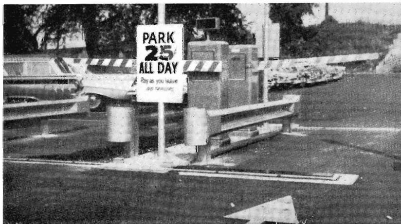
**A** commuter parking lot at Matheson, Illinois, has automatic gates installed. An approaching motor car trips a treadle to raise the entrance gates; when leaving, the driver deposits a coin to open the exit. Instal-
