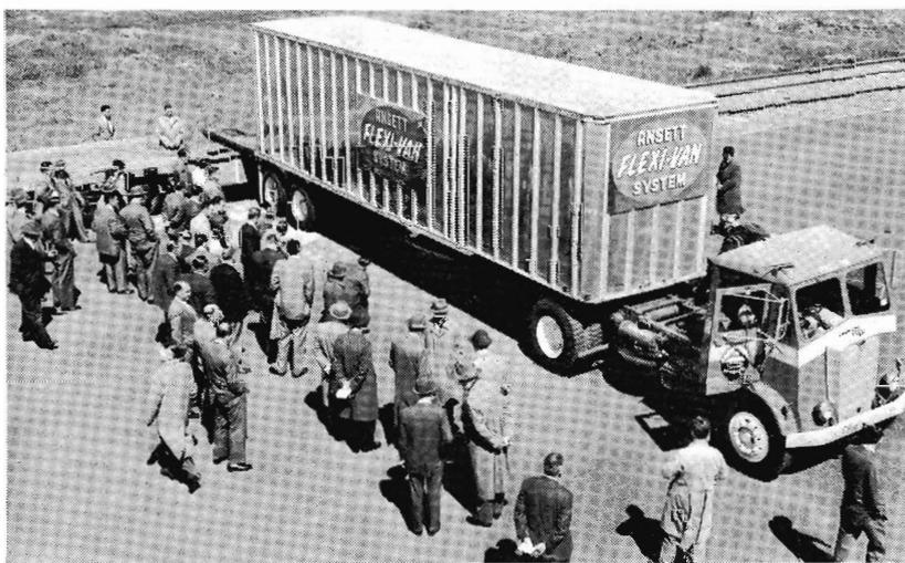
Lining up trailer van body with turntable of rail wagon.
