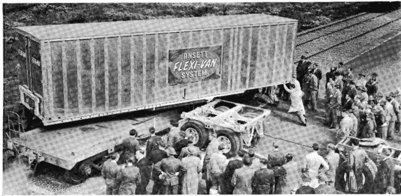
Flexi-van being revolved on turntable to line up lengthways with rail wagon.
