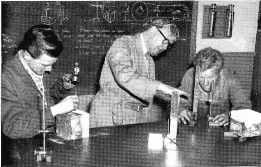
(Above) Apprentice Fitters and Turners N. Parfitt and J. Stevenson being taught by Instructor J. Mitchell in the marking out of a chipping block exercise. (Right) Performing the finishing operation on a "G" clamp is Apprentice Fitter and Turner P. Browning.
