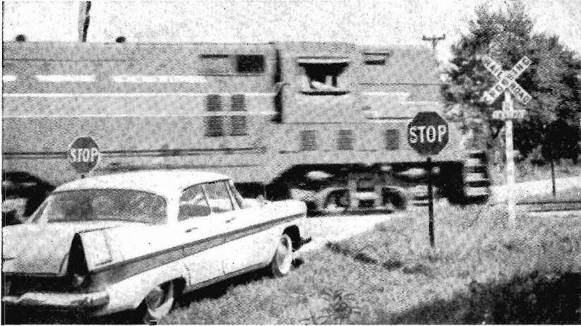
A 75% reduction has been made in the annual number of accidents at 313 railroad crossings of secondary highways in the State of Michigan, U.S.A., by installing red and white octagonal "stop" signs (above) at crossings protected only with the conventional crossbuck signs.
