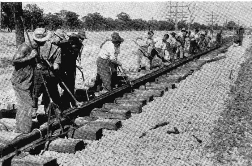
Standard gauge creeps nearer Melbourne. Close to Benalla this 90 ft welded rail is being turned into position after which it will be "pinned" down by the pre-driven dog-spike. In the right of the picture can be seen the metallised edge of the existing 5ft. 3in. gauge track.
