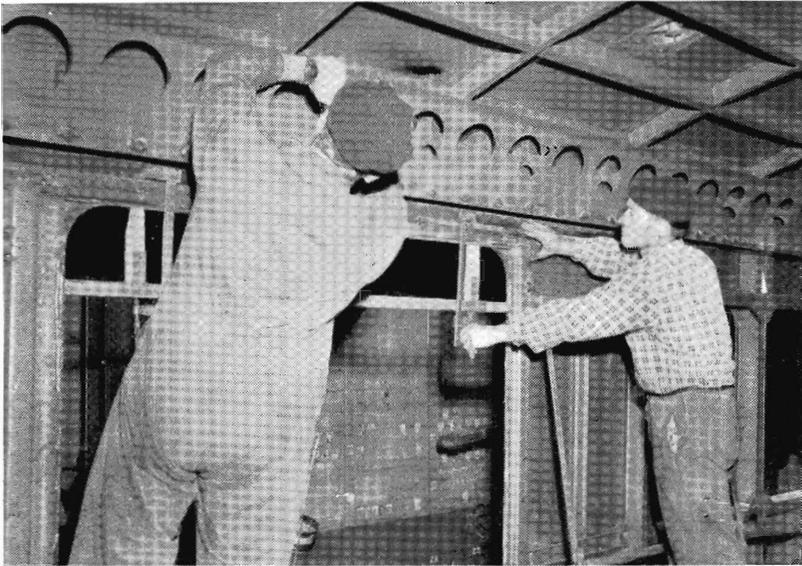
(Above) **COMPLETING** interior of shells before spraying with sound insulation. (Below) T.V. cameramen covered the building of the trains, including this work on an underframe in a special revolving jig.
