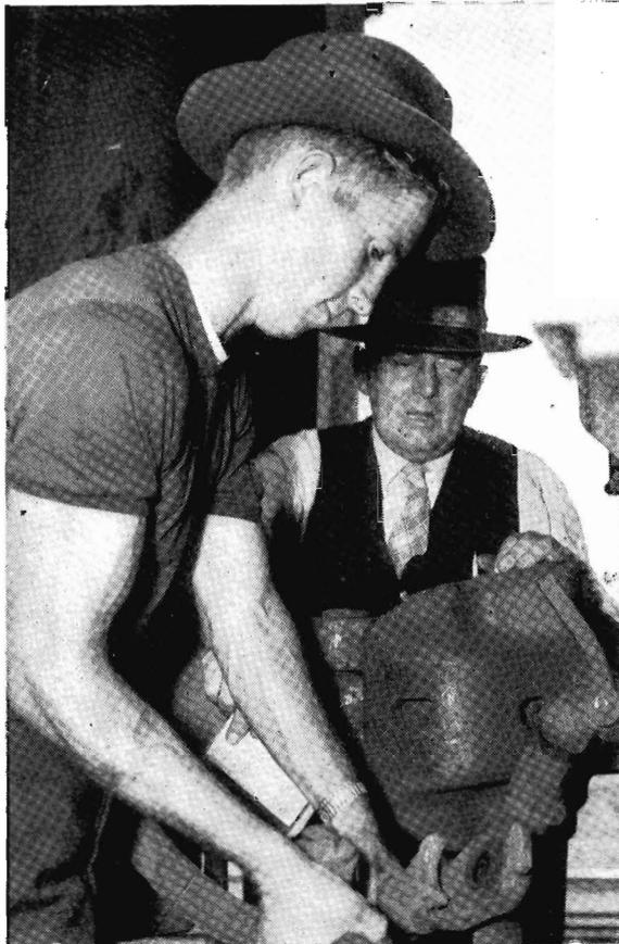
Symbolizing the link between the Victorian and New South Wales railway systems, N.S.W. Shunter L. Masterson couples wagon air-brake hoses at Albury with Victorian Yard Foreman B. Rook looking on.
