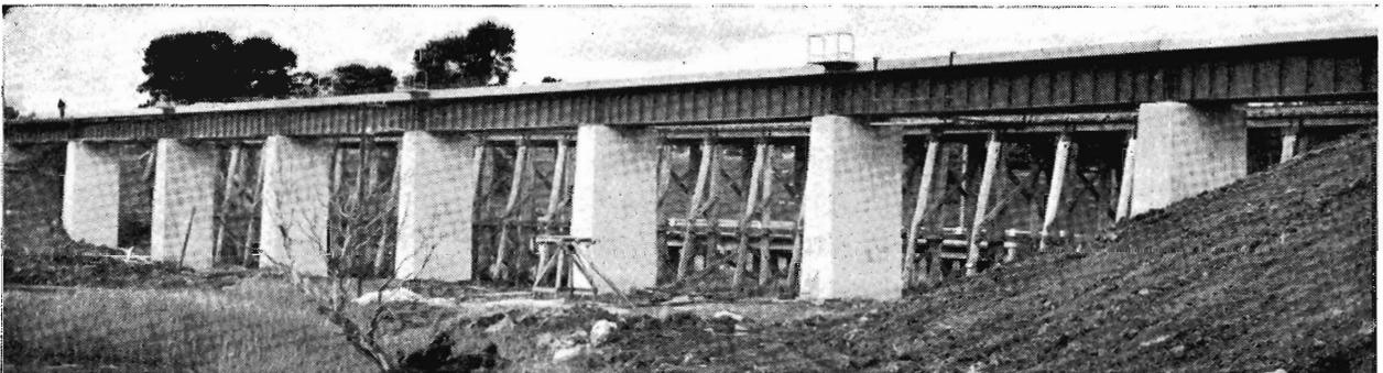
This impressive bridge over Mt. Emu Creek, between Boorcan and Terang, was recently completed by district Way and Works Branch staff. On a new alignment of track, it replaces the old (1887) timber bridge seen in the background. With eight 63-foot spans and three of 40 feet, it has a total length of 624 feet. All the piers are founded on concrete shell piles, some going down to 50 feet. The concrete structure will need much less maintenance than timber. (Photograph: Warrnambool Standard).
