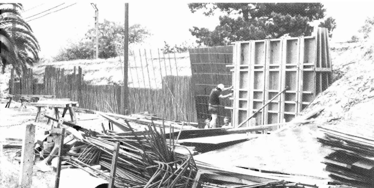
**RETAINING WALL.** A retaining wall is put into position between Ormond and Glenhuntly for the Mordialloc third track.
