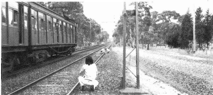
**NEW STATIONS.** Surveyors check measurements on the site of the new station, between Noble Park and Dandenong. So far only the ballast has been laid so that the tracks can be shifted to allow for the island platform. Between Seaford and Frankston—the site for the other new station approved for construction—new track has been laid and will be shortly joined to the existing track. When this is done the tracks next to the front-end loader will be removed to make way for the station.
