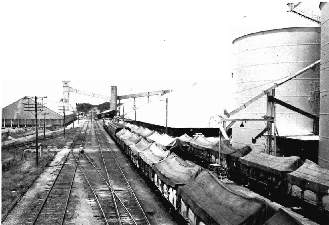
Wheat trains wait to be unloaded at the huge Grain Elevator Board's silos at Dunolly. The silos have an overall capacity to handle 323 700 tonnes of grain. Of this, the silo on the right can take 272 100 tonnes, the two local storage bins at front right 3 900 tonnes, and the silo on the left 47 700 tonnes. Dunolly receives grain to meet export and local requirements.
