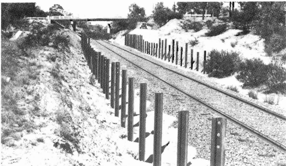
**BUANGOR:** Supports in place for sheeting a cutting as part of a stabilisation programme. Stabilisation is necessary in some areas to prevent tracks being covered by sand.
