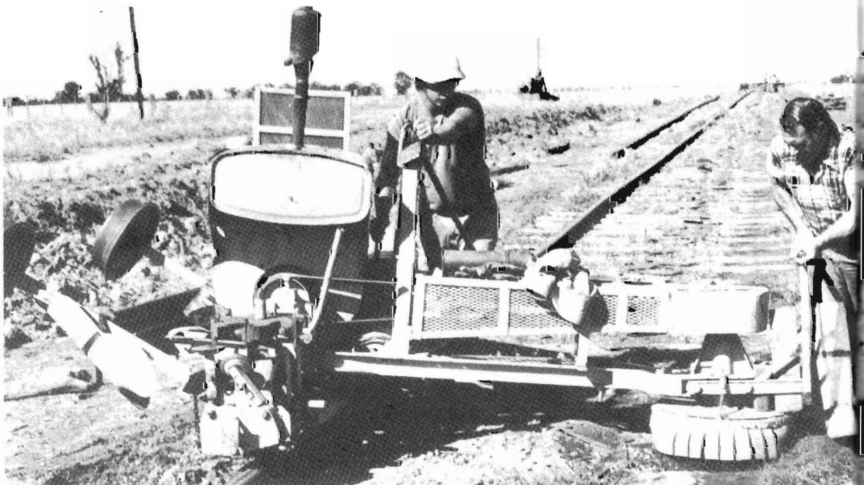
**DENILQUIN - MATHOURA:** A mechanical adzing machine in use during track relaying operations. The machine is guided on one rail as it trims the other side of the sleepers before the second rail is spiked in place.
