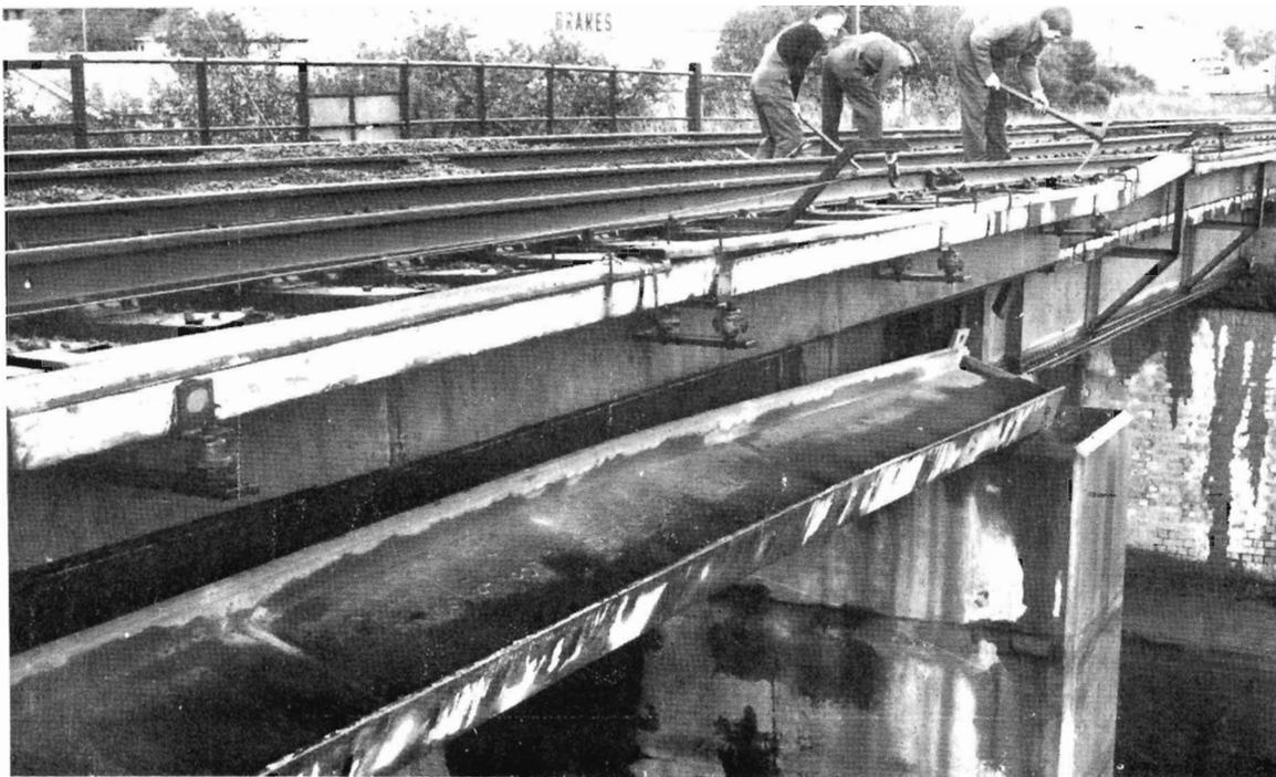
Victorian Railways staff make urgent track repairs after a truck has hit and damaged a bridge at Wantirna. Immediately above the displaced girder, signal cables have only just escaped damage.
